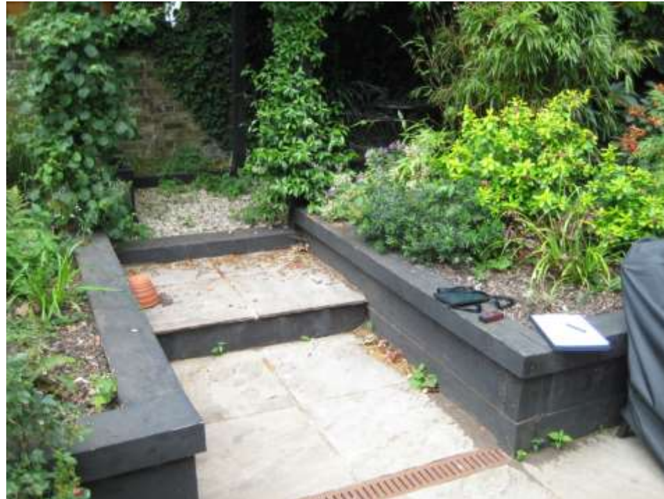
Fig X – It appears that the rear garden ground level has previously been raised. This was most likely undertaken when the rear extension was added.
