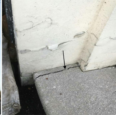
Damage to front steps at main entrance
