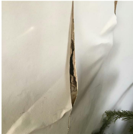
Crack in Flat 28 living Room
