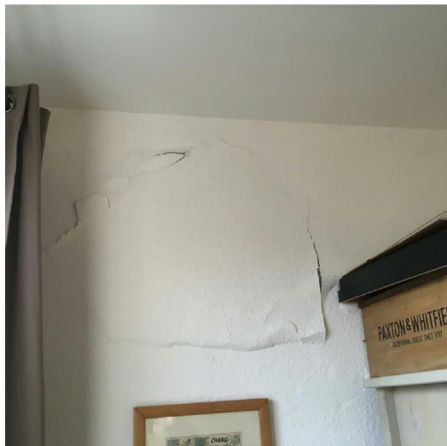
Cracking in Flat 28 Right hand end bedroom
