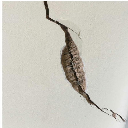
Close up of crack in the entrance lobby showing evidence of past repair
