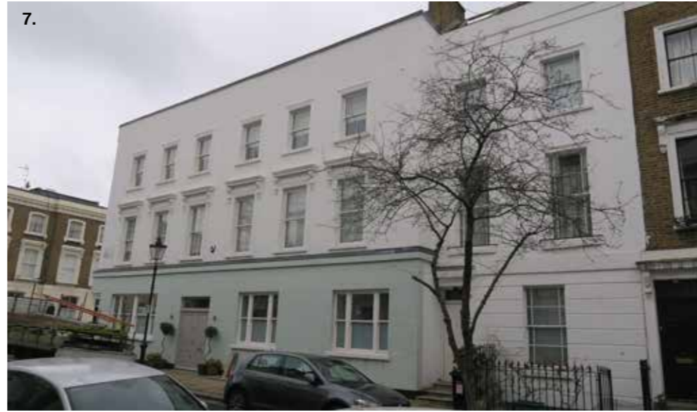
7. Three-storey side extension (possibly original) at the corner of Chalcot Road & Edis St. (North Side).
