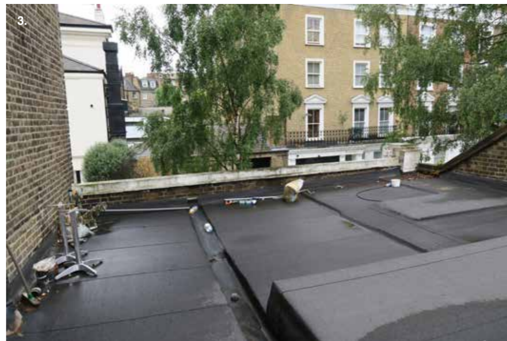
3. View from the roof of the No.91a Laundromat
