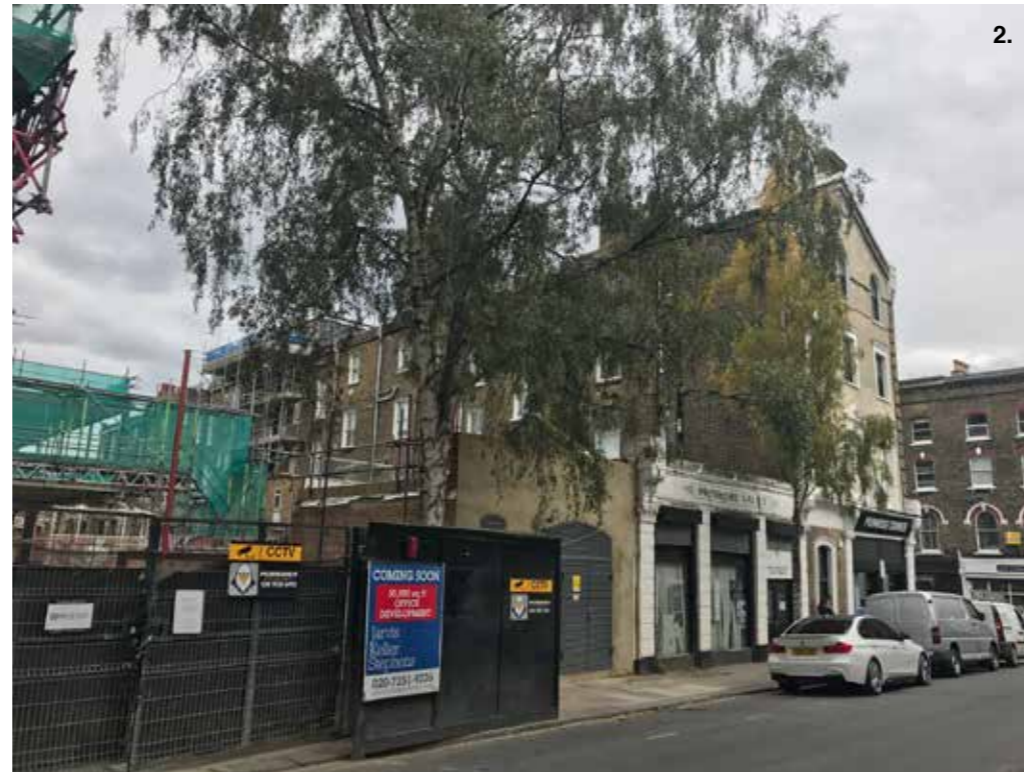
2. View through the gap to the rear of Nos.91-109.
