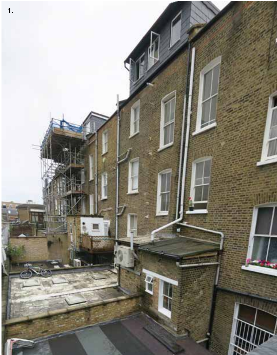
1. View of the rear elevations to Nos 93-109 Regent's Park Road
