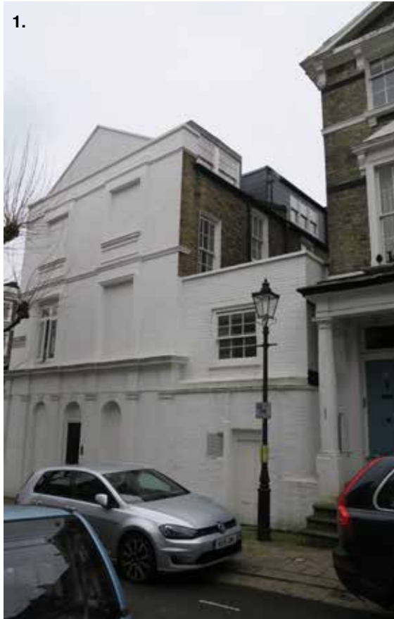
1. Two-storey infill side extension (possibly original) at the corner of Chamberlain Road & Regent's Park Road (North Side). The gap between the buildings is fully infilled.
