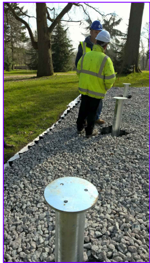
Images of screw pile installation
