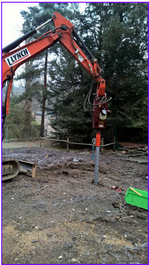
Images of screw pile installation
