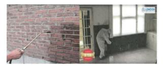
Salts contained in water are absorbed into the masonry and subsequently into the plaster coat, these appropriate specifications will prevent any residual salts in the base substrate migrating into new plasterwork.
