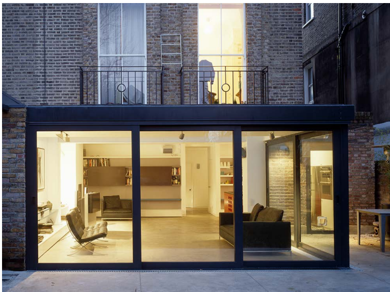
Picture 2b: Aluminium frame glazed doors maximise light
