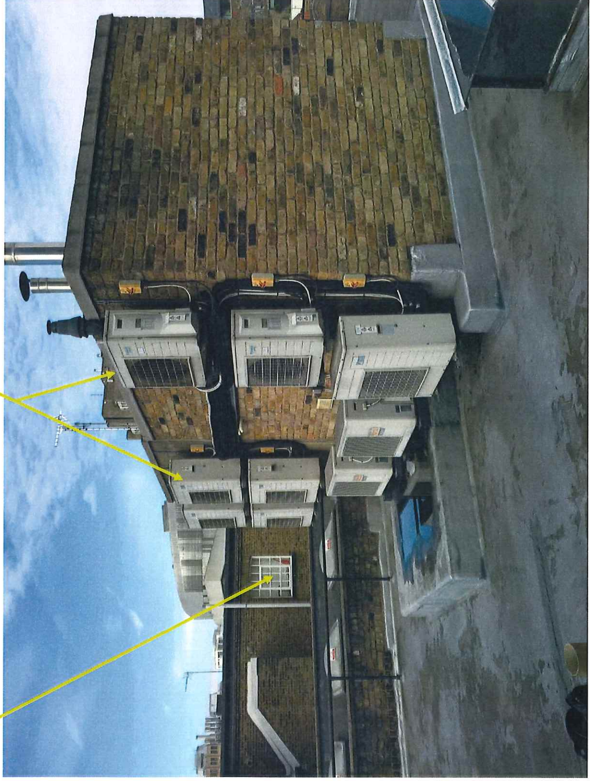
Photo G – View of Existing AC Condensers Fixed to Roof Plantroom with Residential Flat's Window Behind
