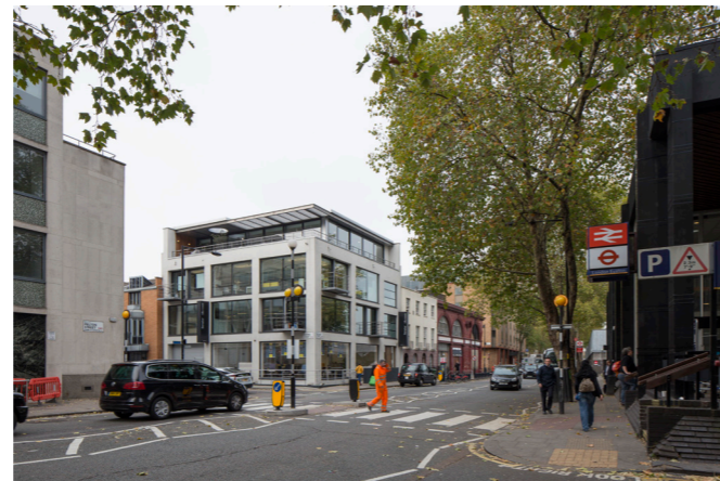
VIEW D MELTON STREET/EUSTON STREET JUNCTION LOOKING NORTH WEST TO IBIS HOTEL
