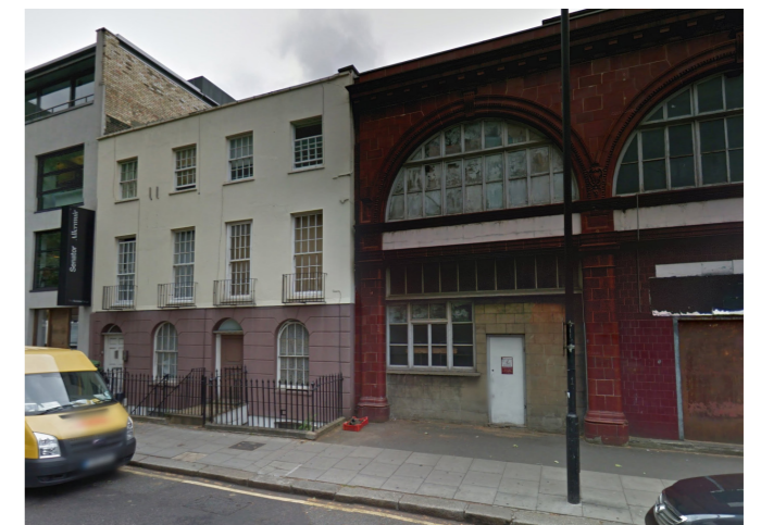
NO'S 14-15 MELTON STREET
