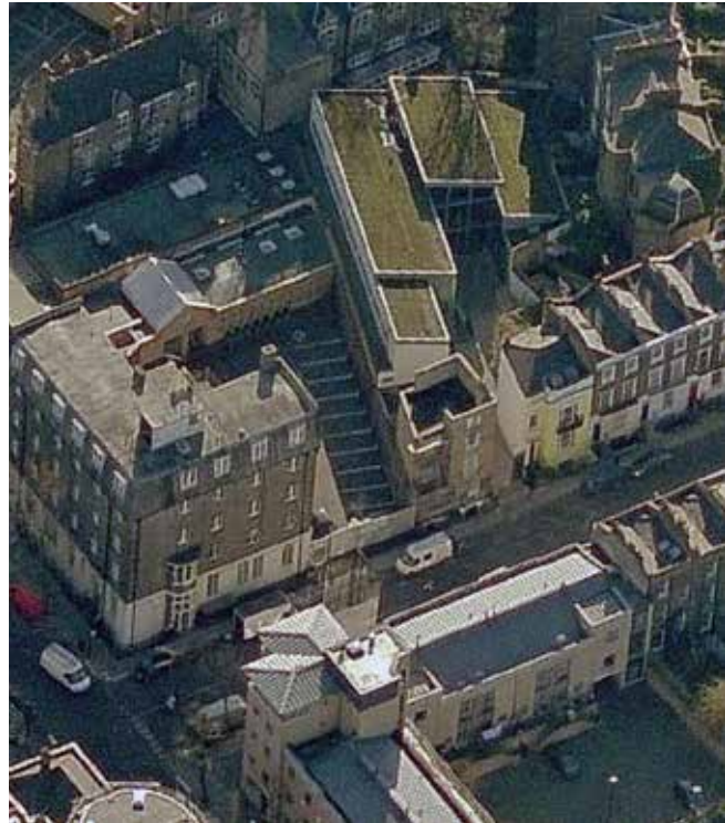
fig 6. Aerial view of 33 Inverness Street + surrounding context prior to the construction of the Cavendish School Building to
