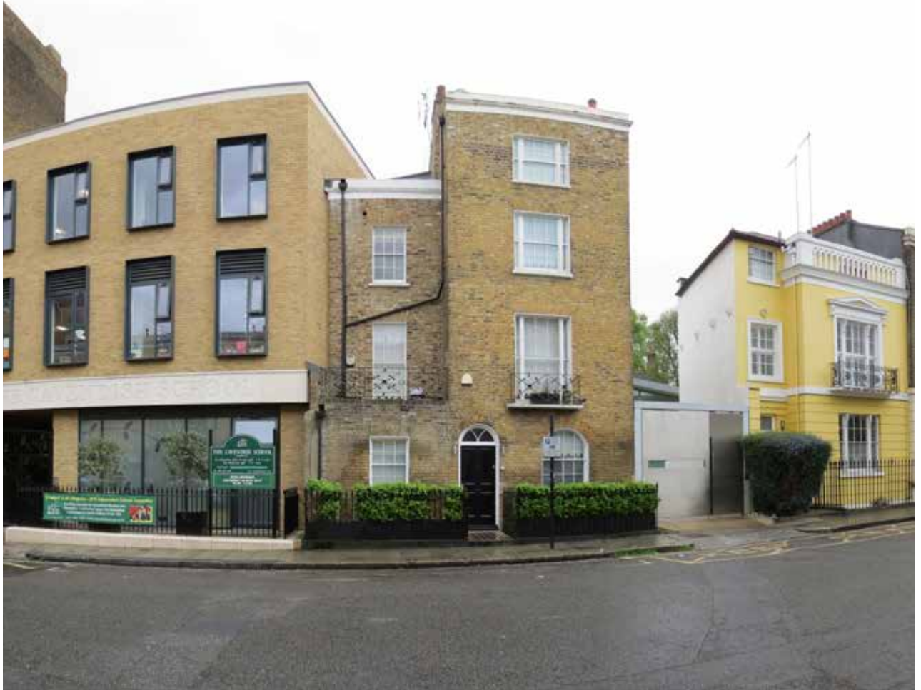
fig 15. 33 Inverness street + neighbouring buildings
