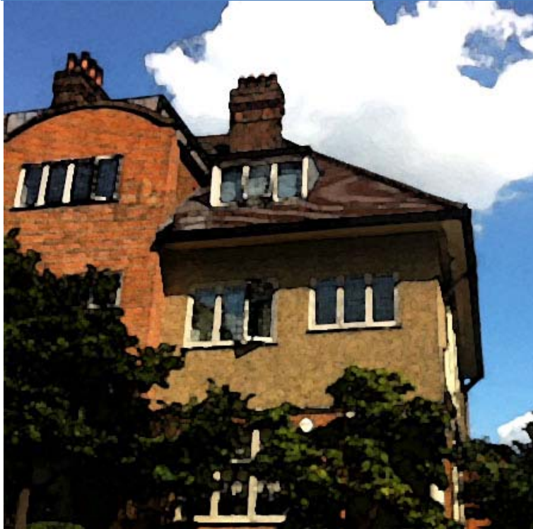
Image 1 Front elevation of property from road
