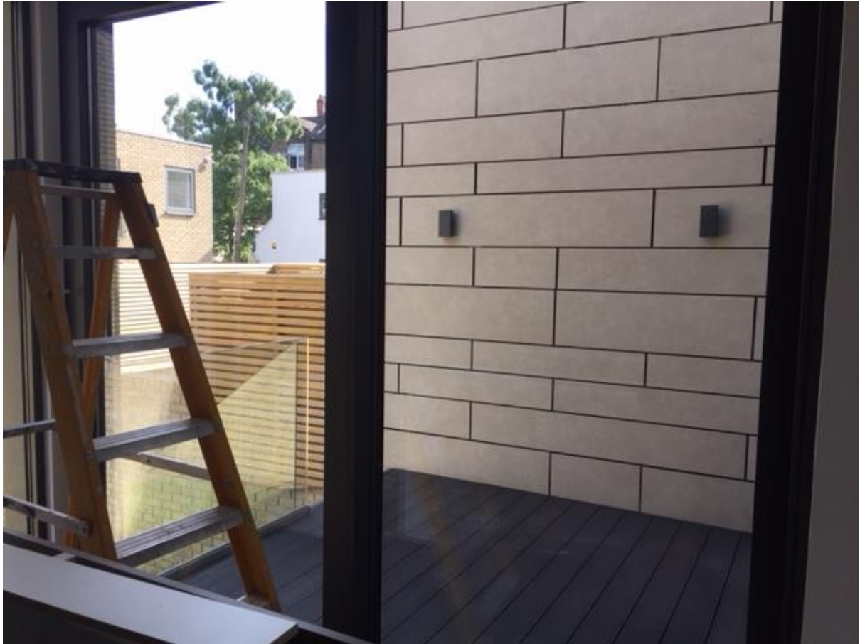
Photo.2 View from kitchen looking over existing terrace with the new Studio apartments and College Lane in the background.
