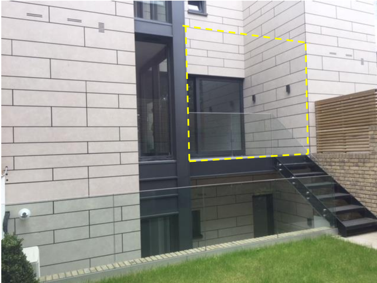
Photo.3 View back towards terrace indicating area of in fill extension.
