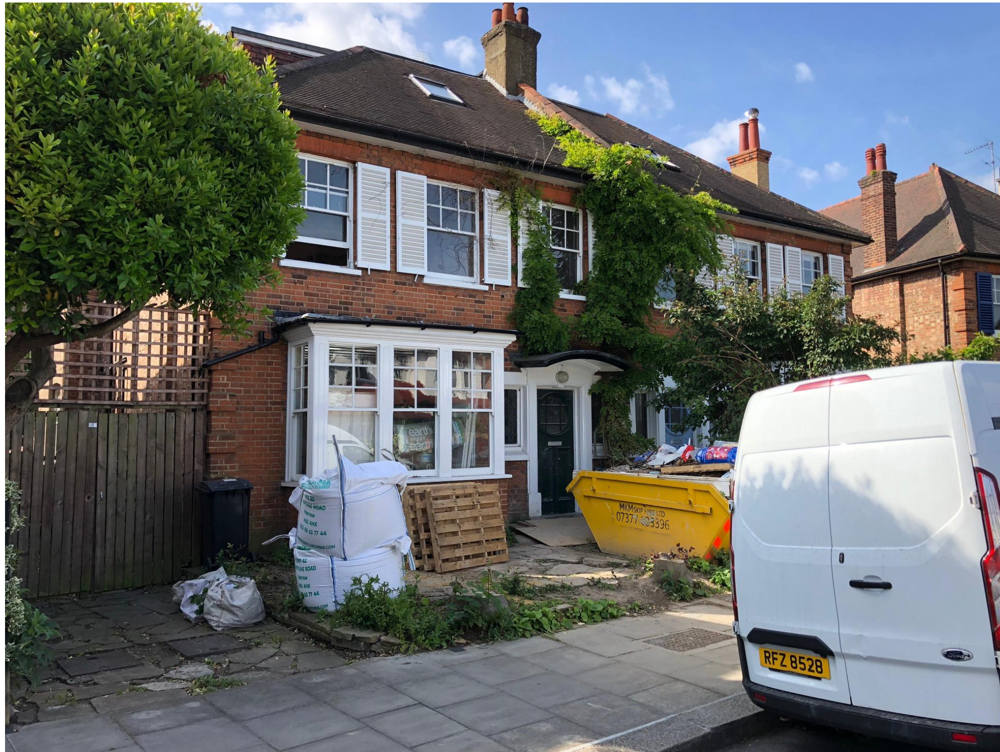
View to the South west detailing the front of the property
