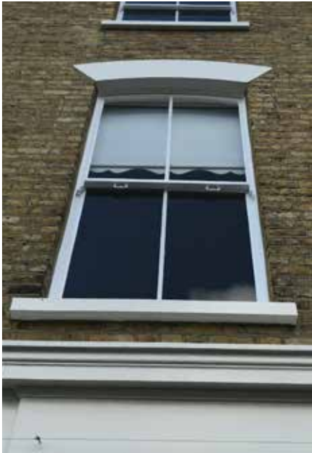
Existing timber sash windows
