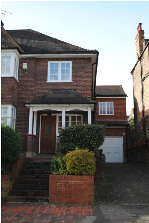
Image of No. 72 Lawn Road - Part single part two storey side extension
