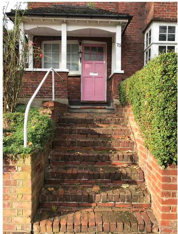
View 5 – Front entrance steps and porch
