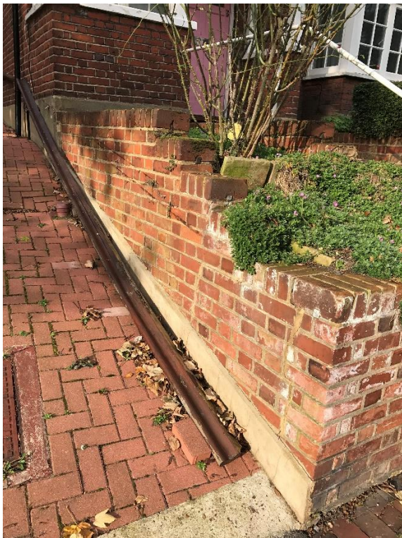
View 4 – Garden retaining wall
