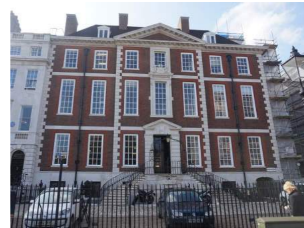
Newcastle House - D
