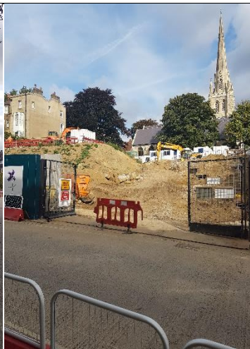
Access to construction site (17 apartments) on New End
