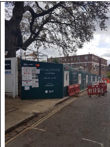
View along New End including construction site
