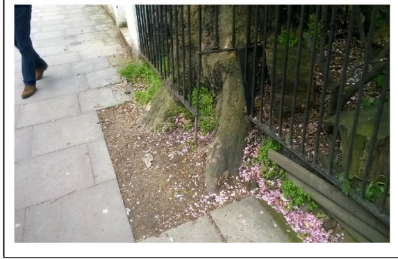
Tree Protruding into Public Footpath
