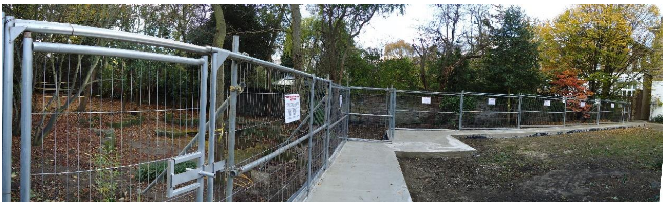
Figure 7. Photograph to illustrate installed protective fencing and ground protection
