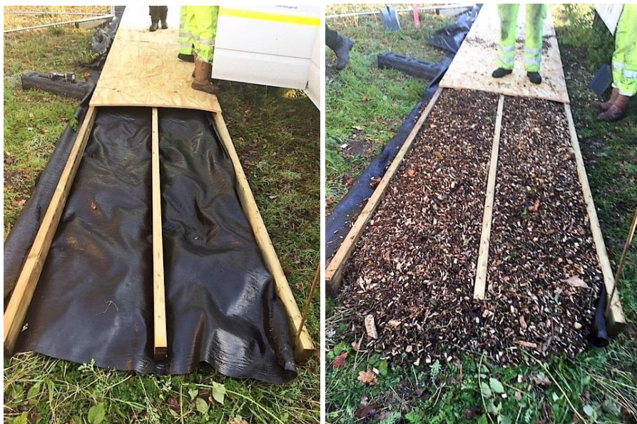
Figure 10. Plywood sheeting used as ground protection.
