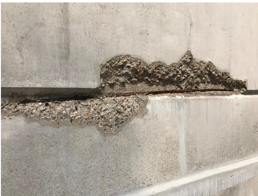
A1.6 South end wall, detail of spalling on east side
