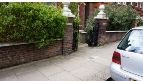
Figure 3: Image of existing front gate posts
