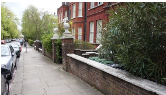
Figure 1: Image of existing front boundary wall
