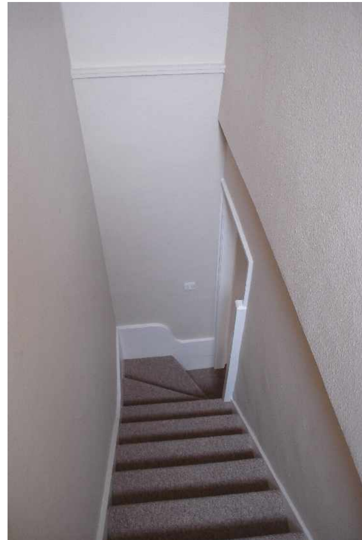
2 nd Floor Stair rising to Roof Terrace
