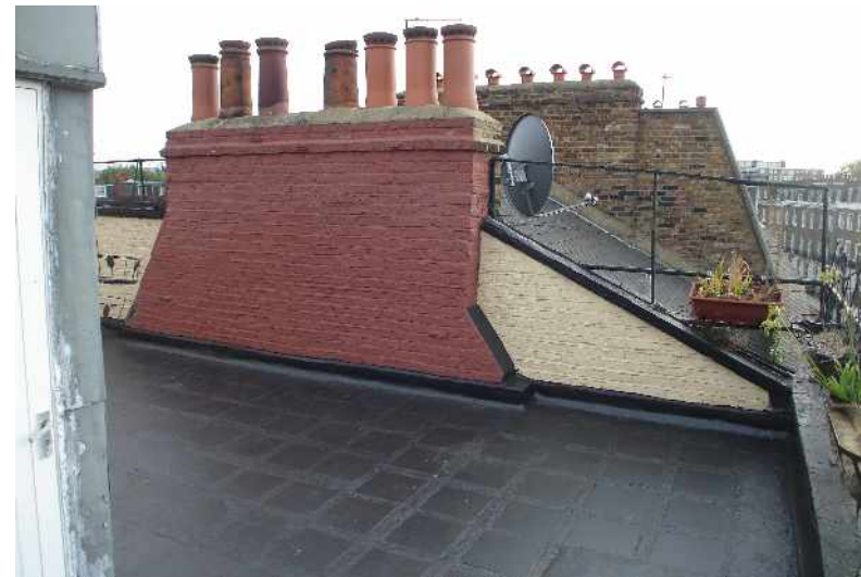
Stair enclosure and Roof Terrace Area
