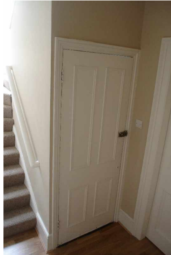
Entrance Door to 76B at 1 st Floor Level
