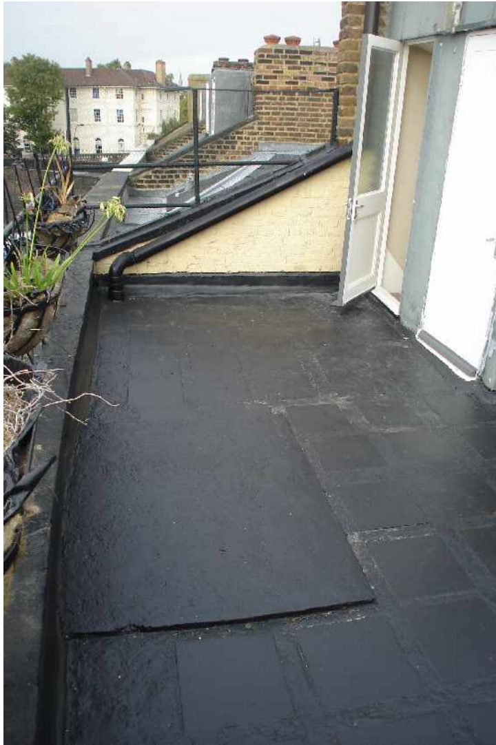
Roof Terrace – Front of Building
