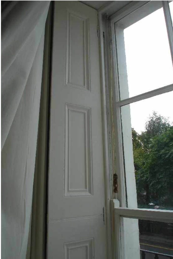
1 st Floor Front Room – Shutters to Windows Retained
