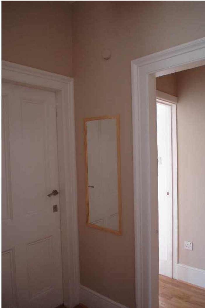
1 st Floor Landing looking through ex'g opening to Front Room
