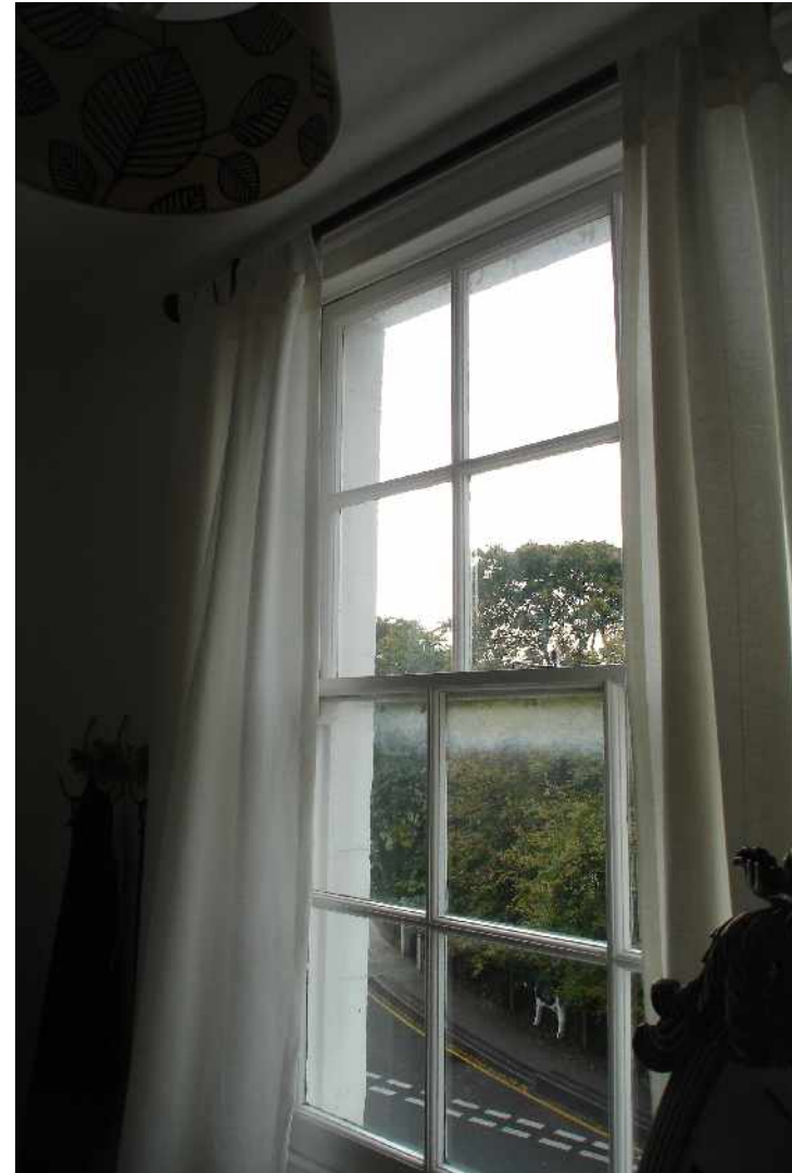
2 nd Floor Front Room – Existing Timber Sliding Sash Windows
