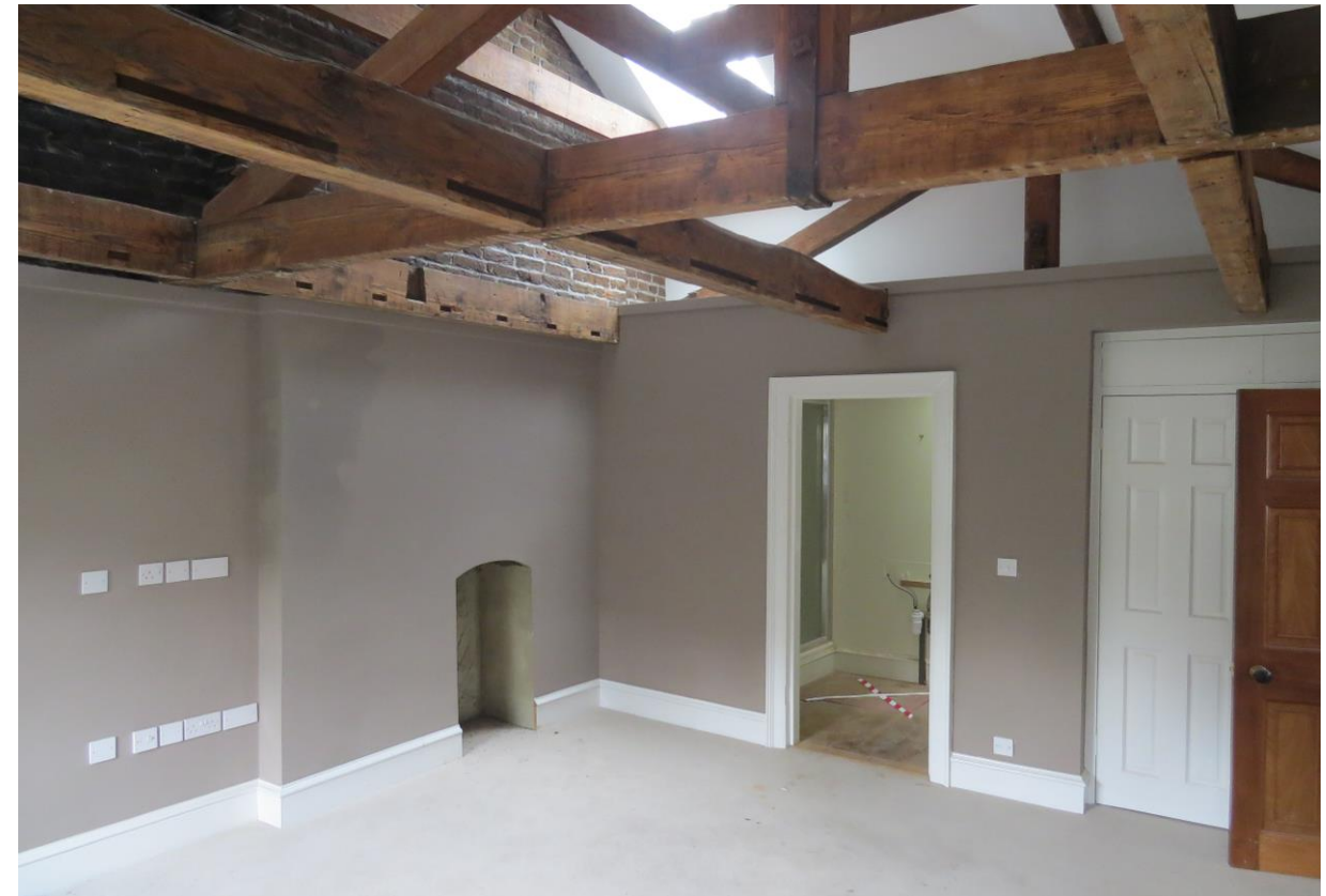
Fig. 25. Third floor rear room.
