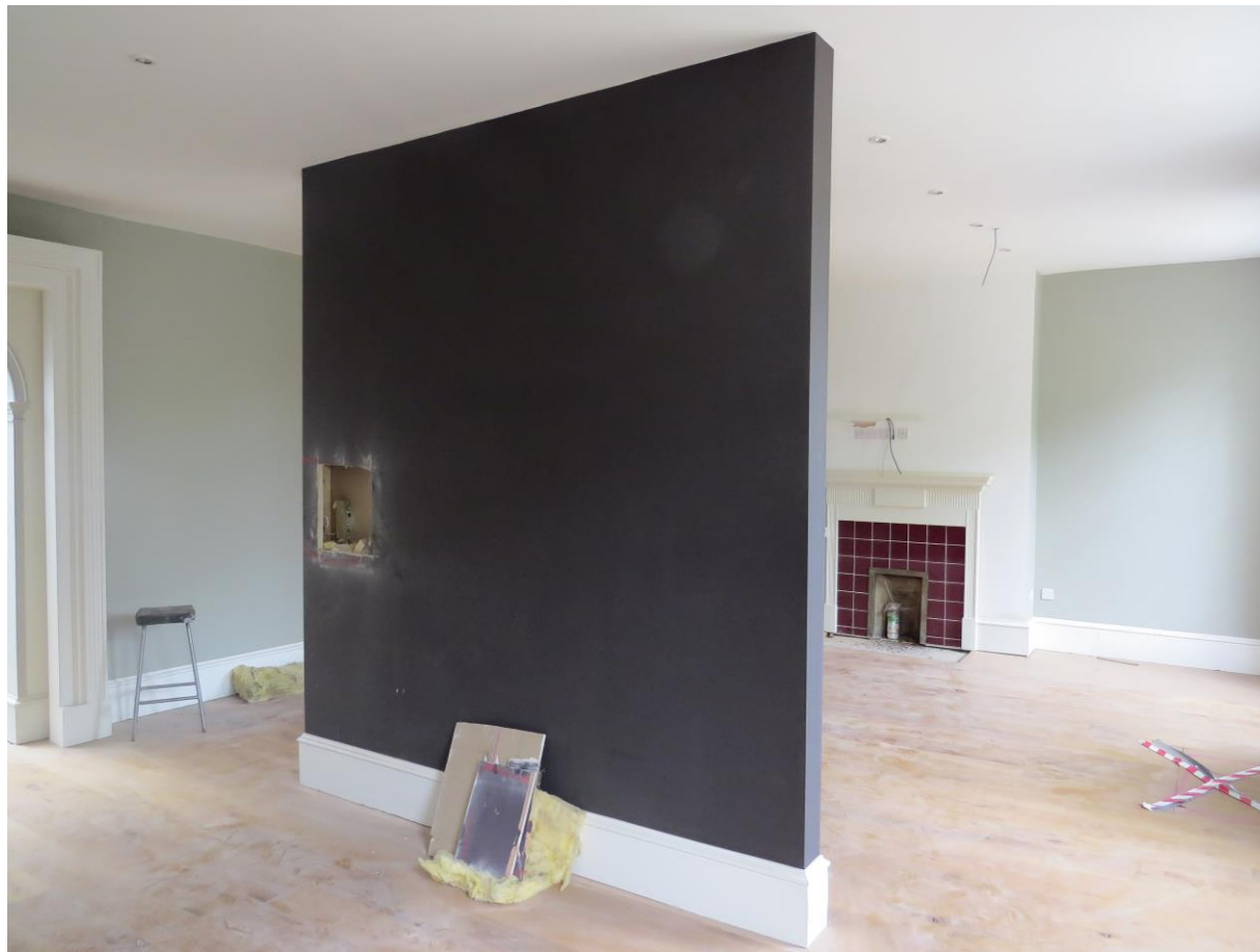
Fig. 23. Second Floor (front) prior to works commencing.
