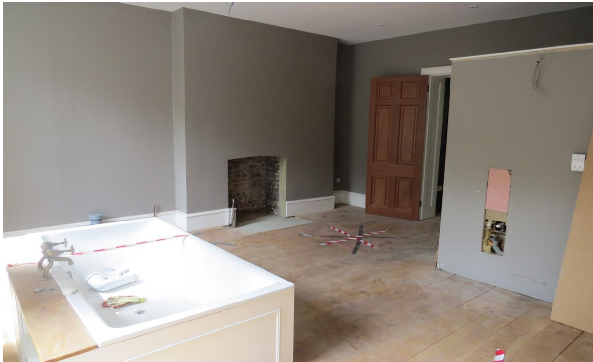
Fig. 24. Second Floor (rear) prior to works commencing.
