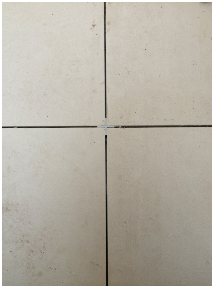
En suite - honed Patara limestone tiles (to be grouted in a colour to match tiles)
