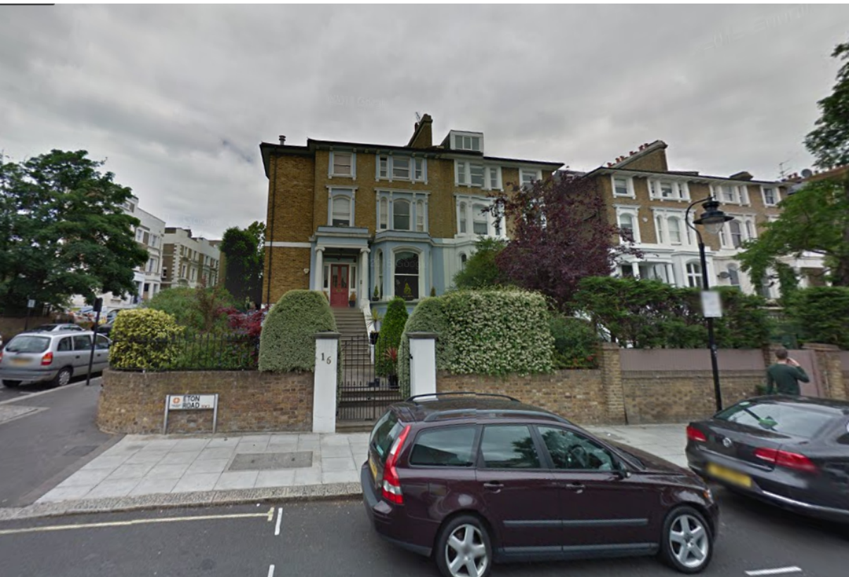
2) Front elevation of no.16 & 18 showing existing dormer at no.18
