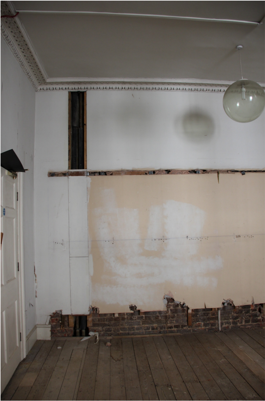
Picture 3 - Ground floor. Vertical pipes into wall void.
