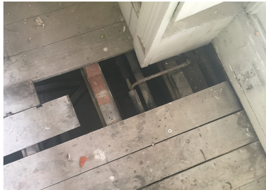
Picture 4 - First floor. Existing radiator pipes and notches.
