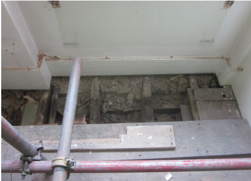
Picture 1 - Ground floor. Existing radiator pipes.
