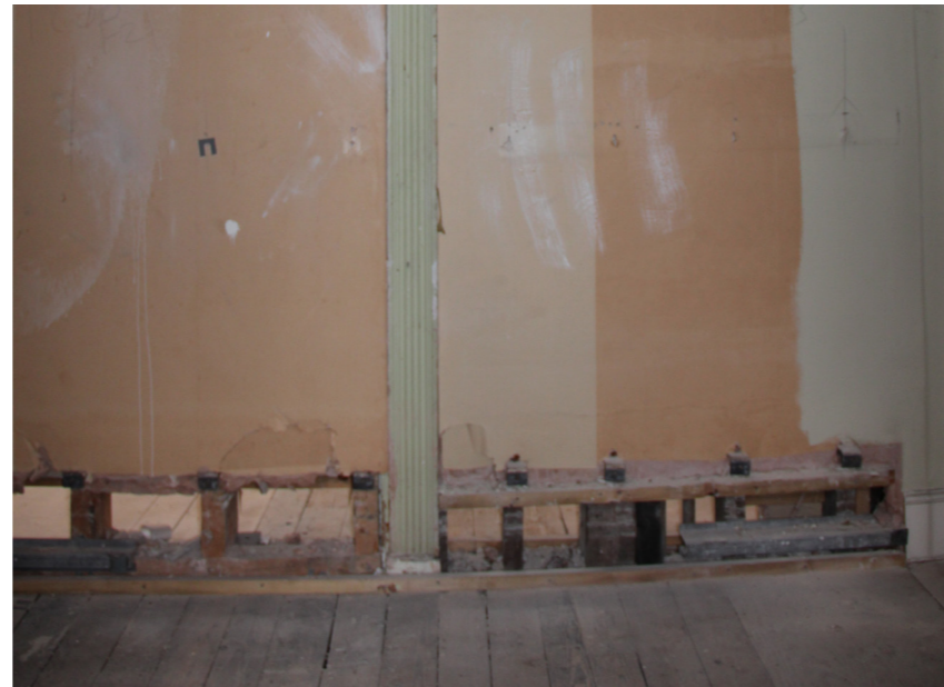
Picture 6 - Ground floor. Vertical pipes into wall void.
