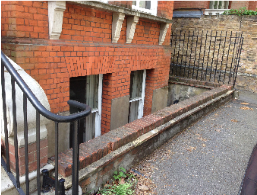
Detail of the one and a half brick high stone sill.
