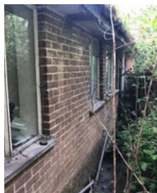
Existing brickwork on the west elevation.
