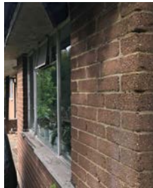
Existing brickwork on the east elevation.
