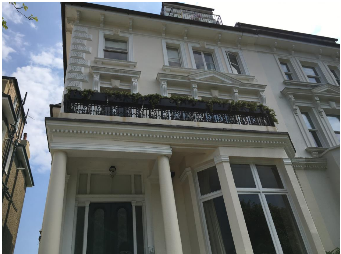
Fig 3: Balustrades to the front of 4E Belsize Grove
