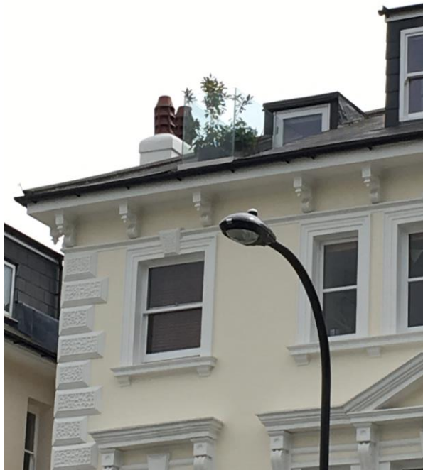
Fig 8: Glass balustrade to front of property in Belsize Park Gardens
