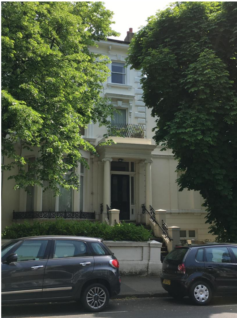
Fig 2: Frontage to 22 Belsize Grove
