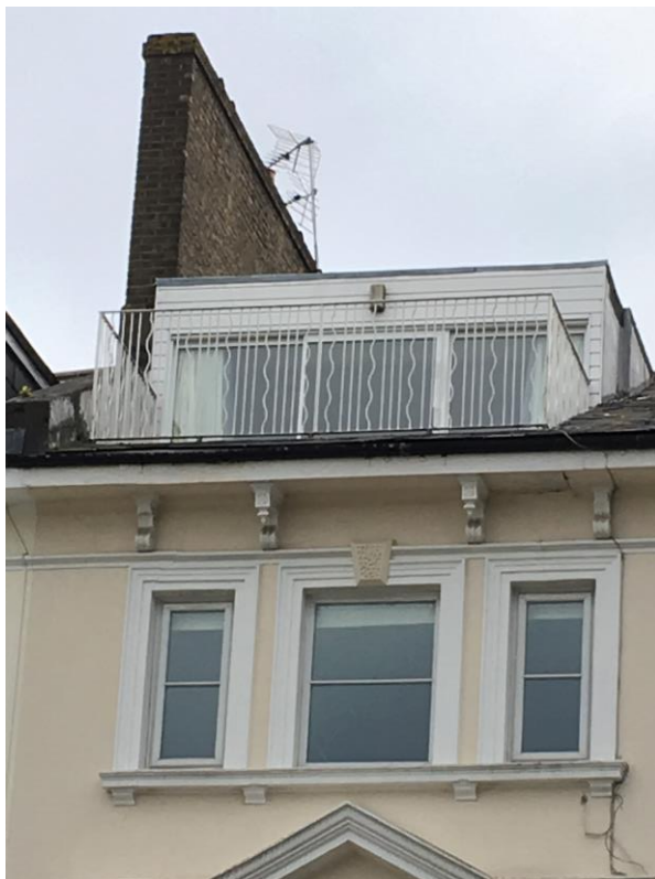
Fig 7: Balustrades to the front of a property in Belsize Park Gardens.
