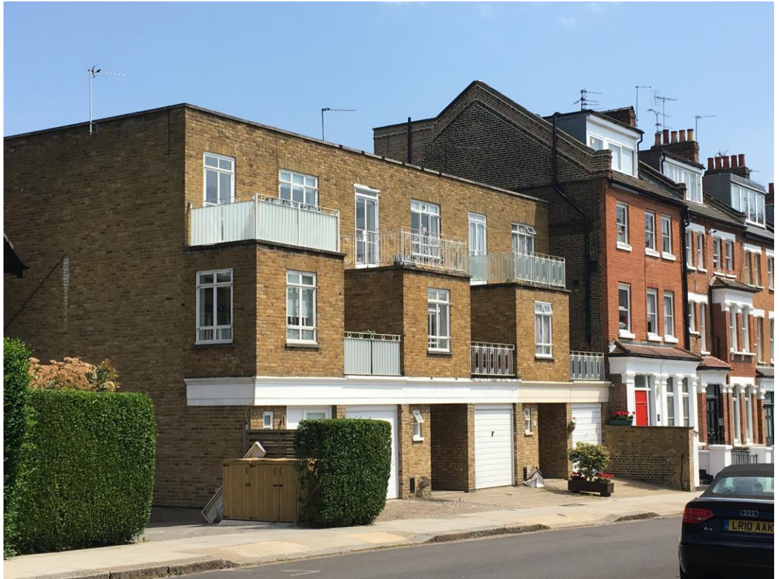
Fig 6: Balustrades to a block fronting Primrose Gardens
