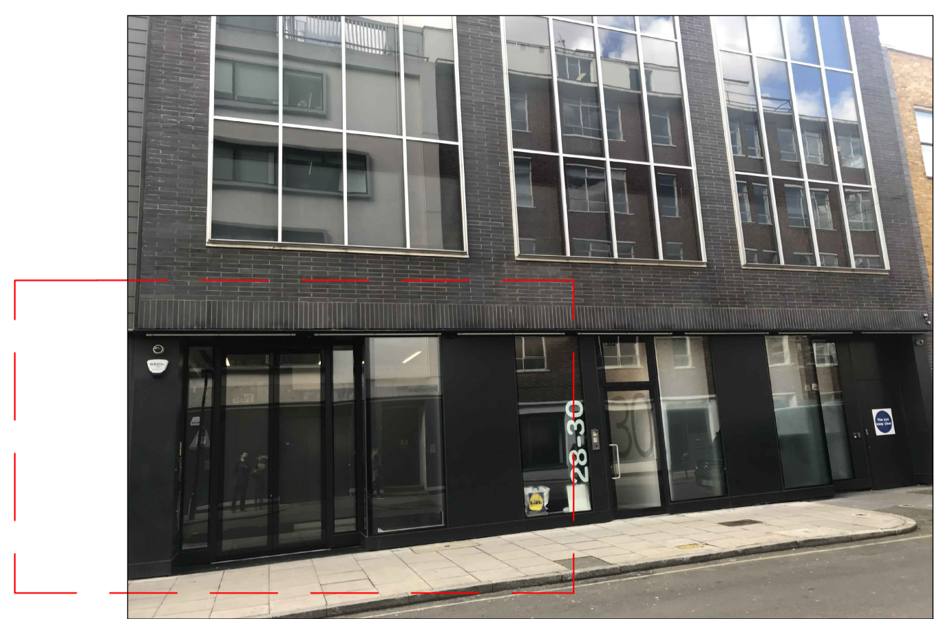
EXISTING FRONT ELEVATION PHOTO SCALE 1:50
