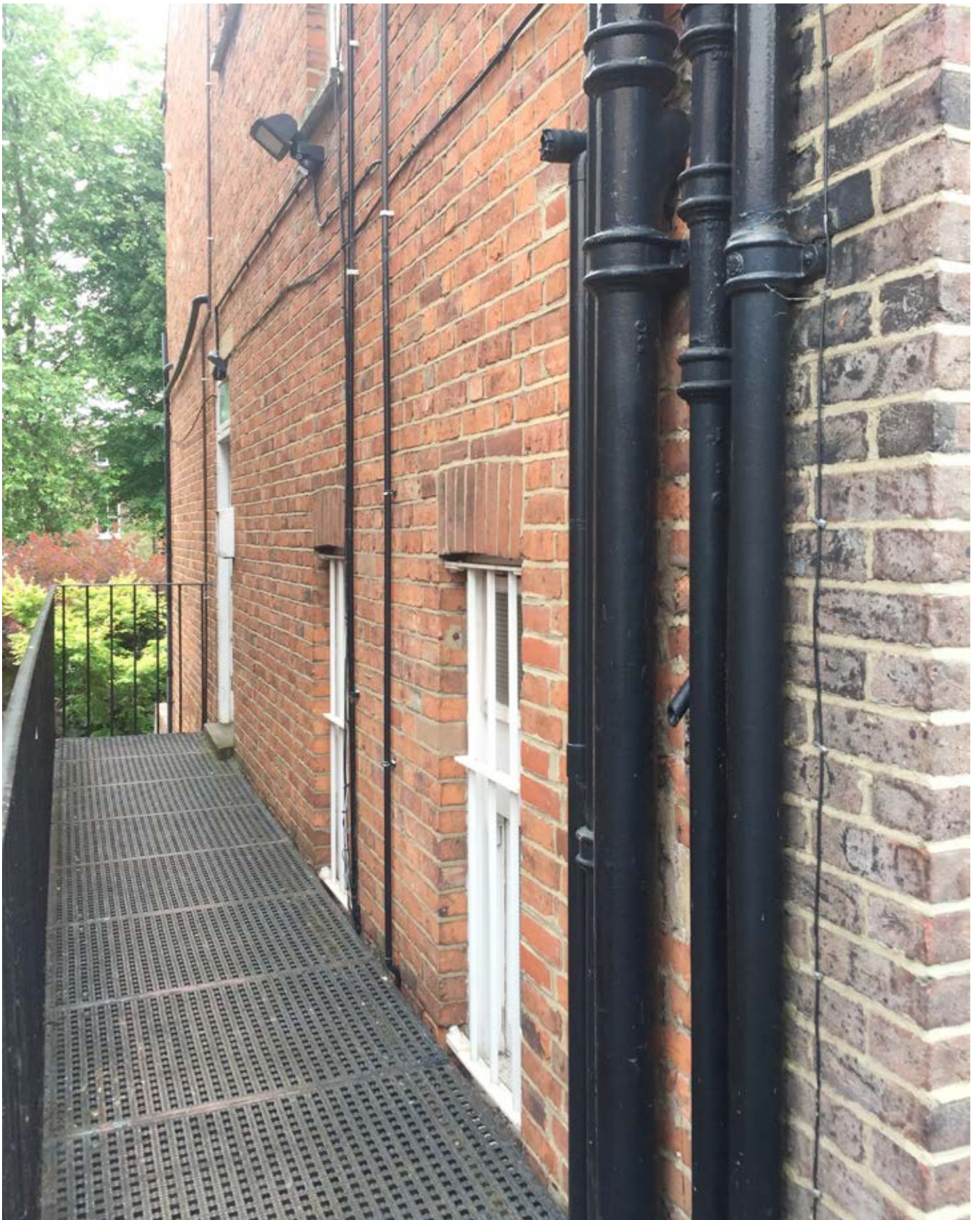
7- Existing suspended metal passageway giving access to flats A & B
