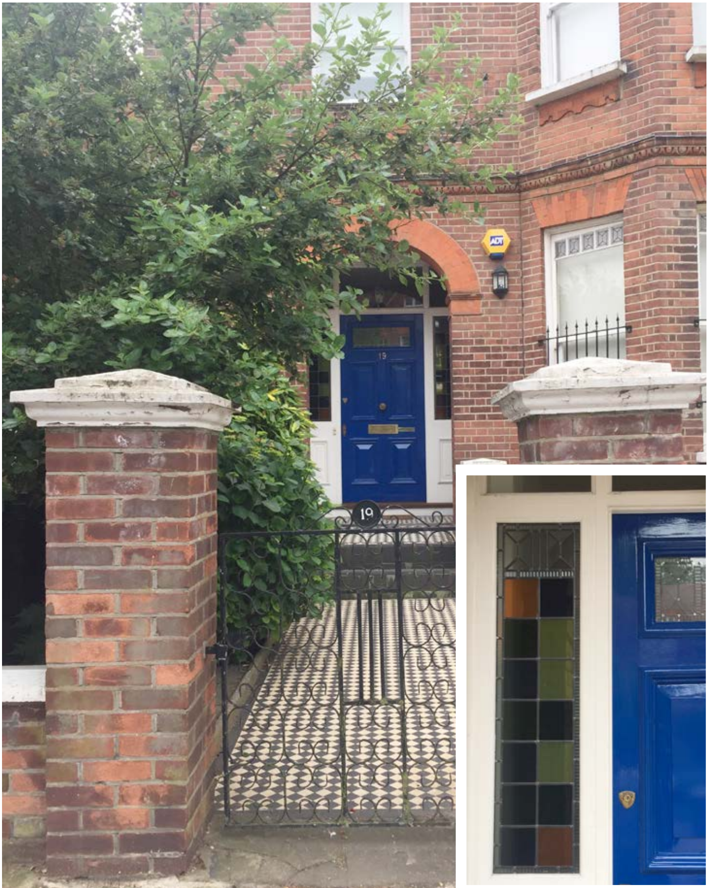
5 - Existing main entrance with metal gate and access door to ground floor flat. The main access the flat has colored glasses on top and sides of the door as per detail on the right.
