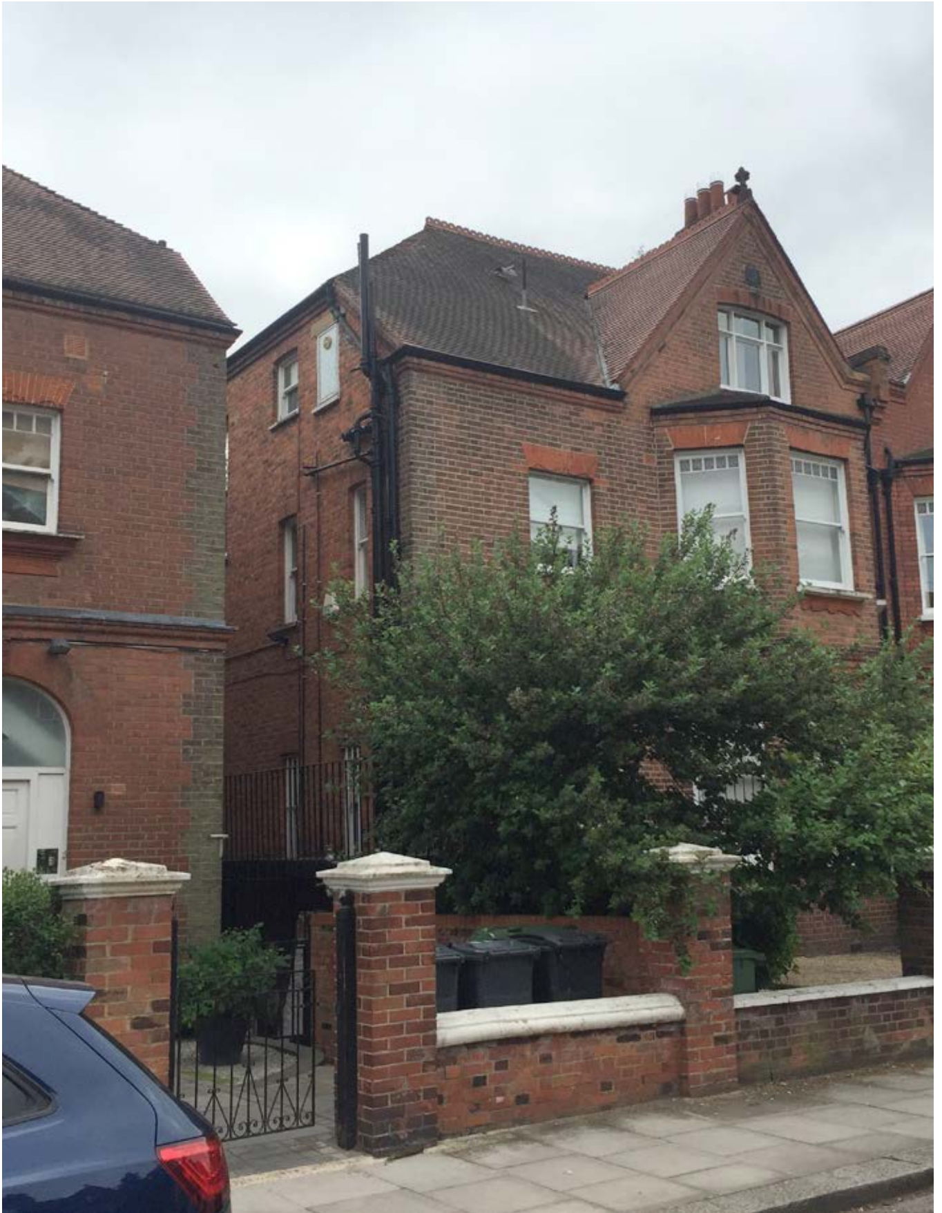
6 - Existing suspended metal passageway giving access to flats A & B from the road (Lambolle Road)
