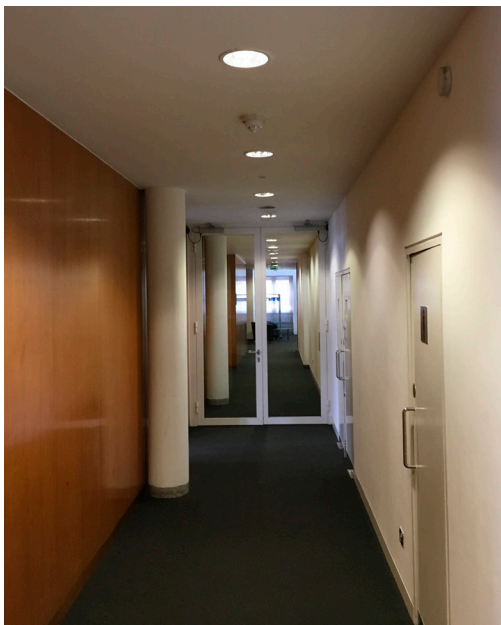
Views of the existing corridor
