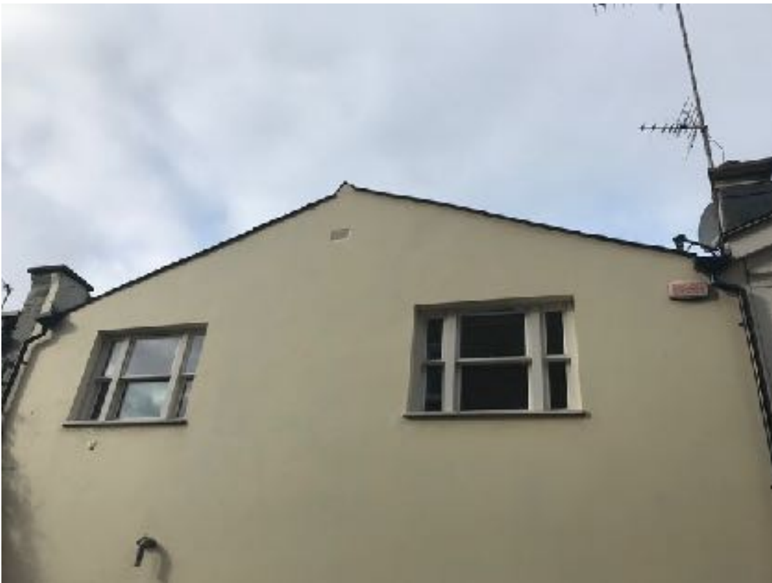
Original shallow overhung slate eaves detail at No 4 which would have been typical of the original mews
