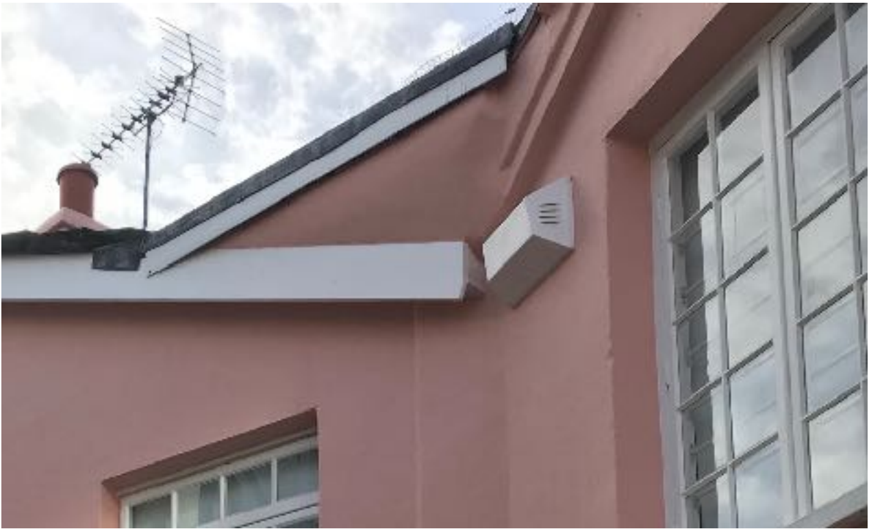
Clumsy roof junction detail
