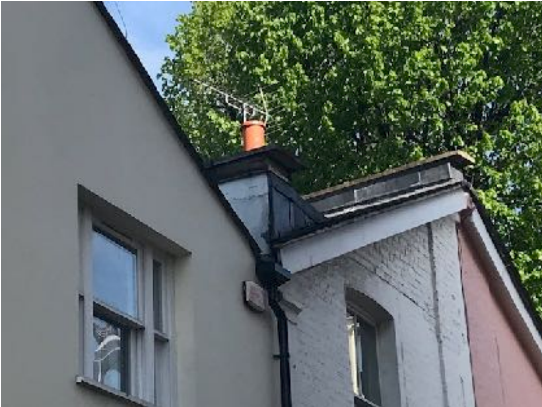
Retained up-stand parapet wall between No 4 and No 5 Albert Terrace Mews
