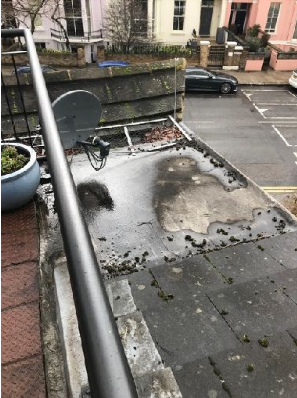
Clumsy roof junction detail from above
