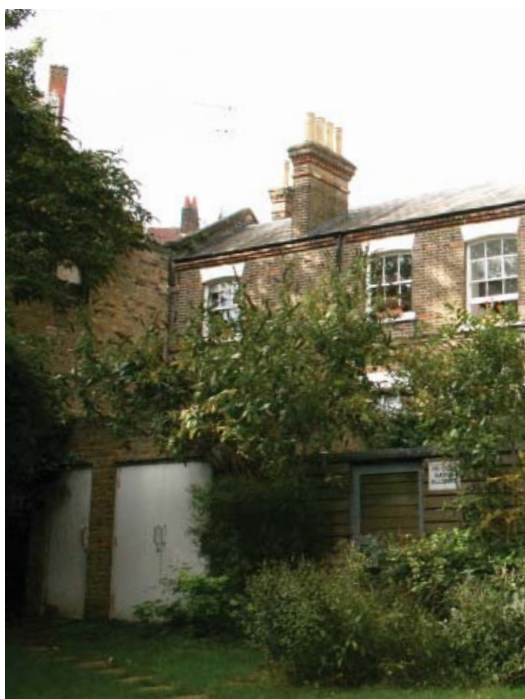
View of substation from New Court Garden
