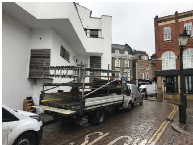
Scaffolding delivery along Back Lane
