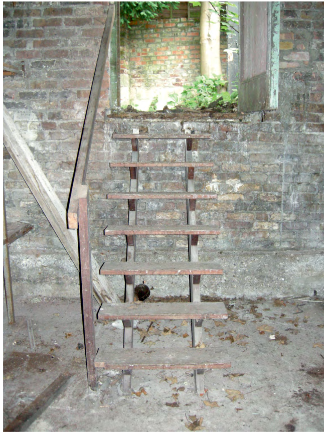
Fig 15 View from north-east of south-west wall of store in north corner of 6 Streatley Place showing depth of floor below ground level (MOLA Photo 16.06.2014)
