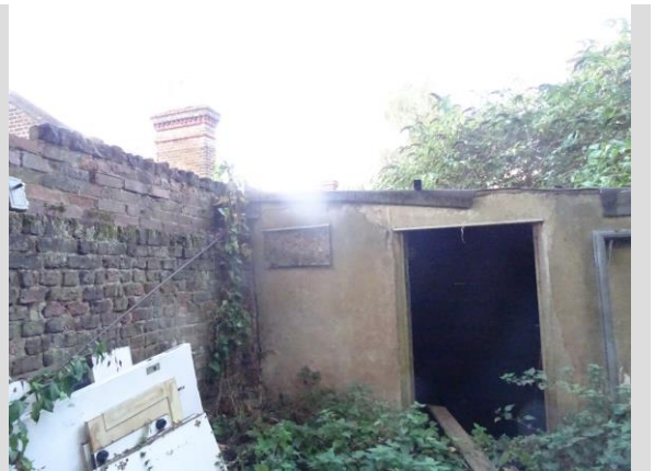
Photograph 4 rubbish dumping over wall
