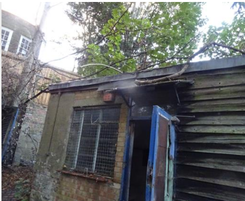
Photograph 3 wooden cladding is too wet and decayed to offer opportunities for heat seeking animals
