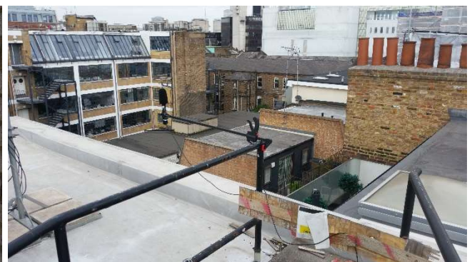
Figure 3.3: Measurement Location 2, close to residential neighbour
