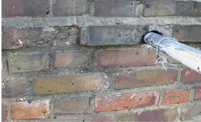
Poorly sealed fixing for handrail
