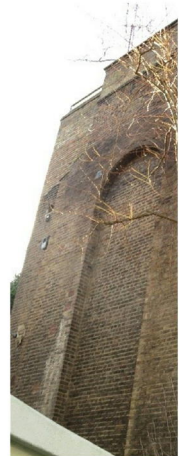
Staining at change of direction of flue
