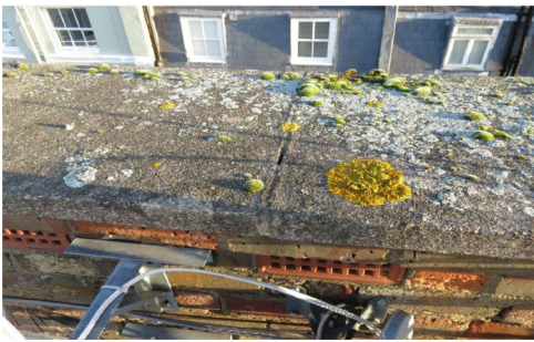
Open joint to coping stone
