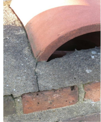
Cracked flue
