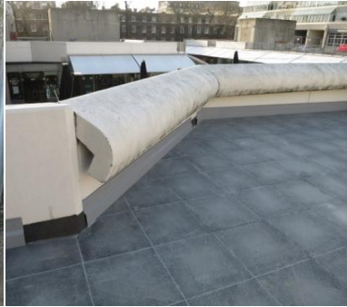
Curved concrete balustrade.
