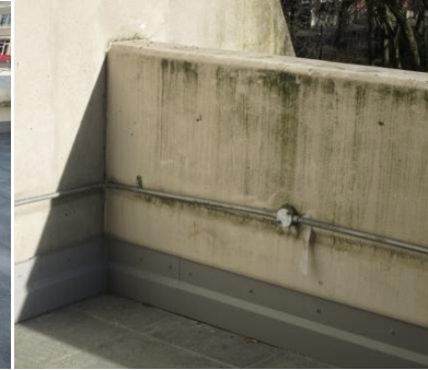
Flat concrete balustrade.
