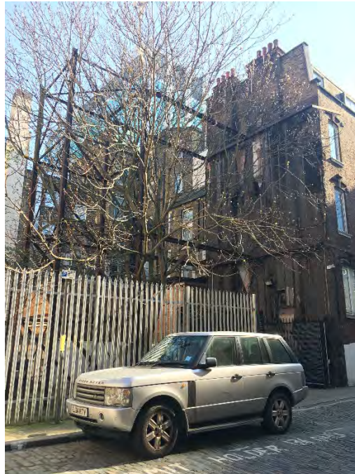
Steel frame structure and mature trees on site
