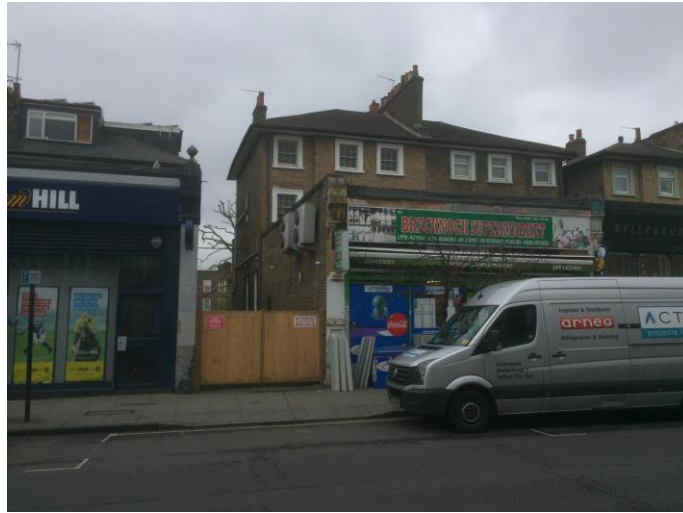
View towards front elevation of 43 Brecknock Road
