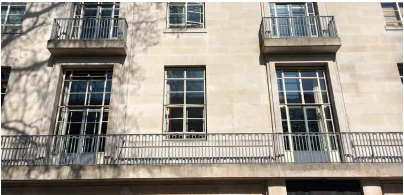
Above_Senate House onto Malet Street showing balustrades to balconies
