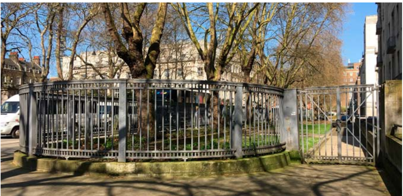
Above_South Elevation onto Montague Place (ADP, 2018)
