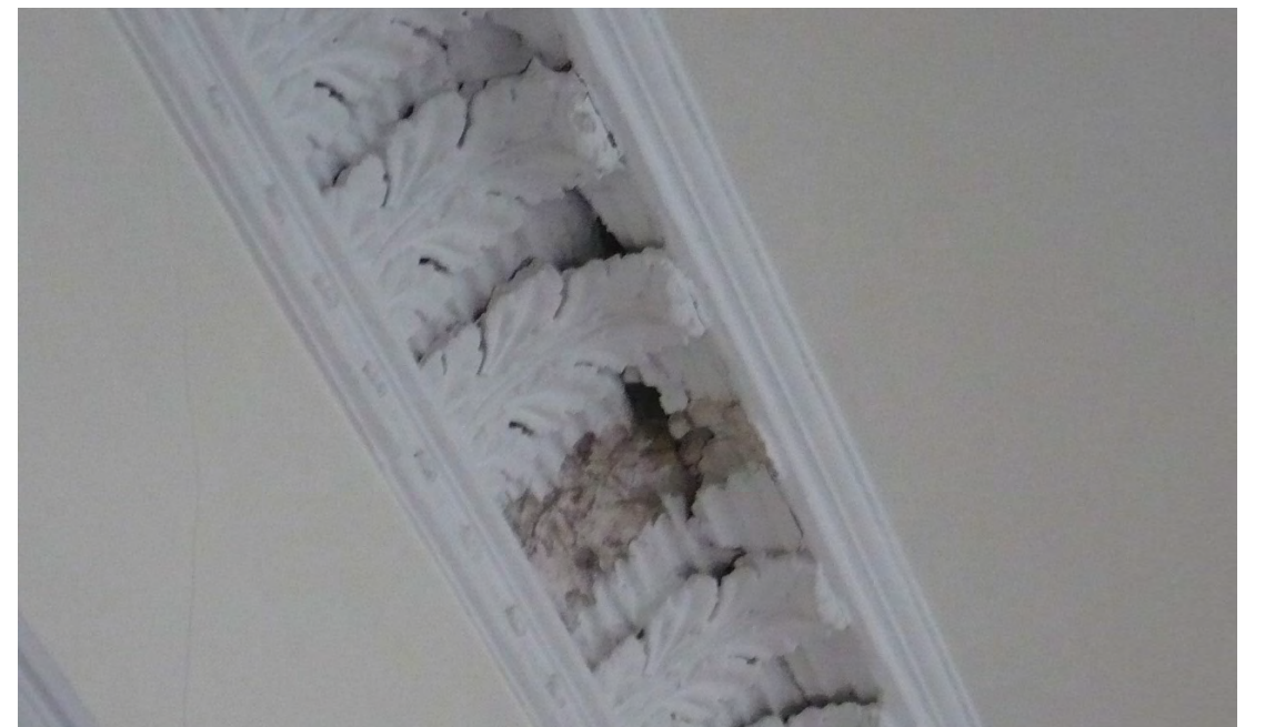
Cornice layered in paint prior to refurbishment
