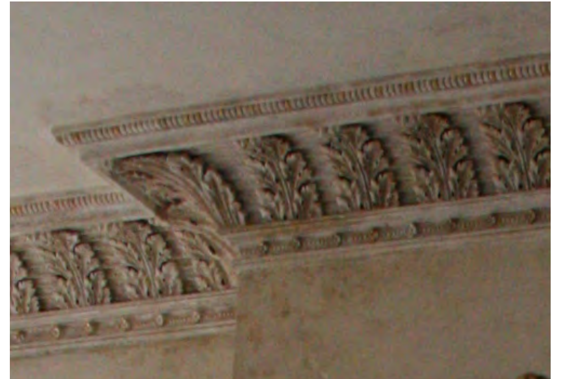
Cornice Stripped back to repair and reveal detail
