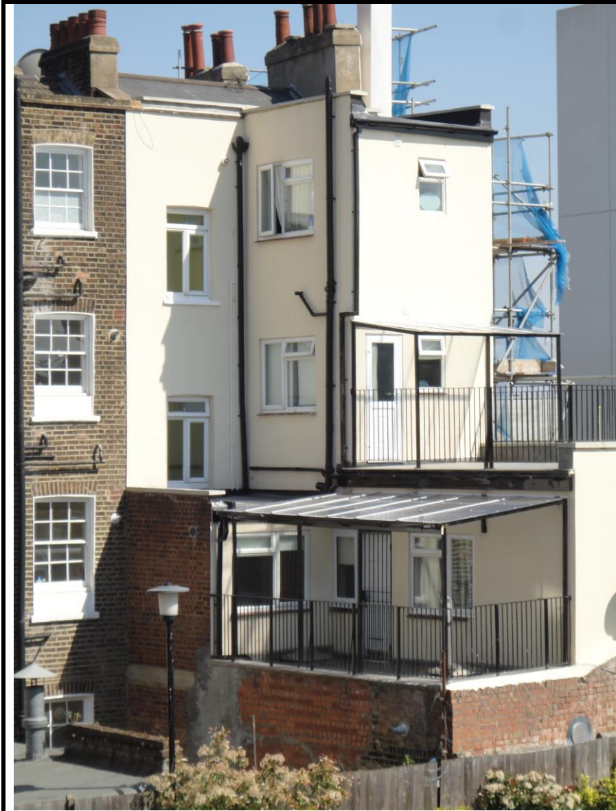
Rear side/rear elevation with canopy and railings creation of roof terrace at second floor level.
