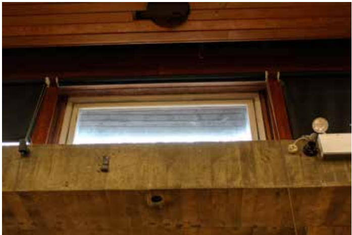
10.3 A close up view of one of the timber clerestory windows.
