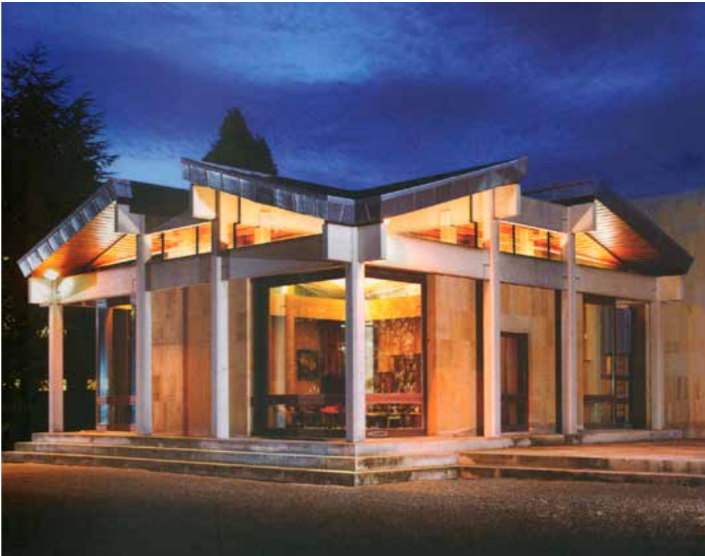
3.4 Downing College, Cambridge, Senior Combination Room, 1965. Note the increasingly confident use of precast elements.
