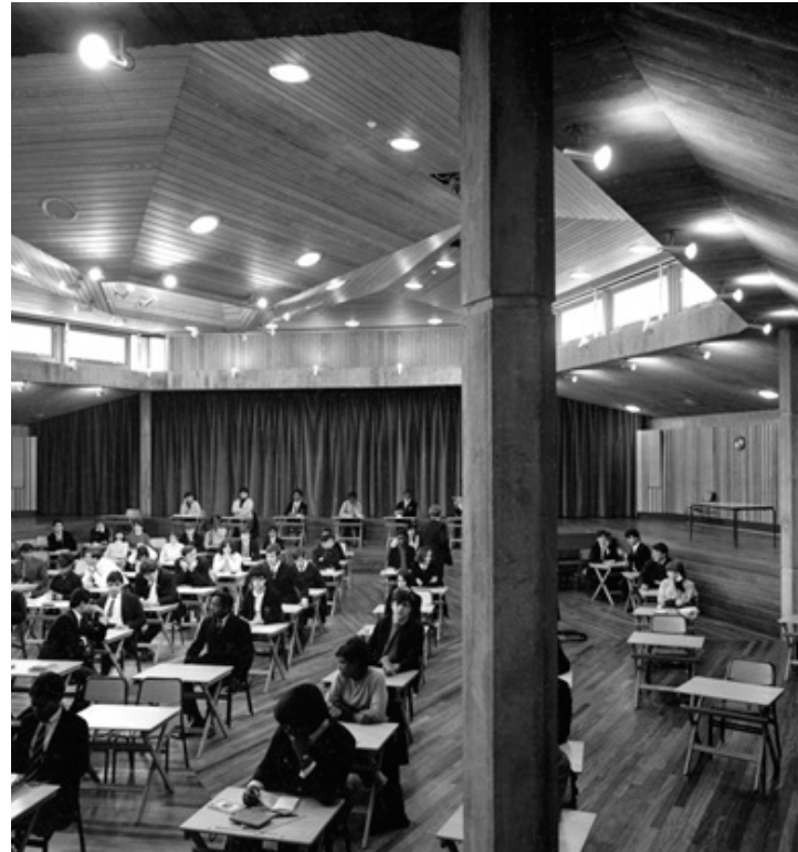
8.2 This photograph shows the main internal volume of the assembly hall. Note the original flush-fitting down lighters integrated into the timber ceiling. These are now sadly lost, leaving behind the empty holes we see today. Also visible are the stainless steel angled lighting to the periphery and the skylight surround.
