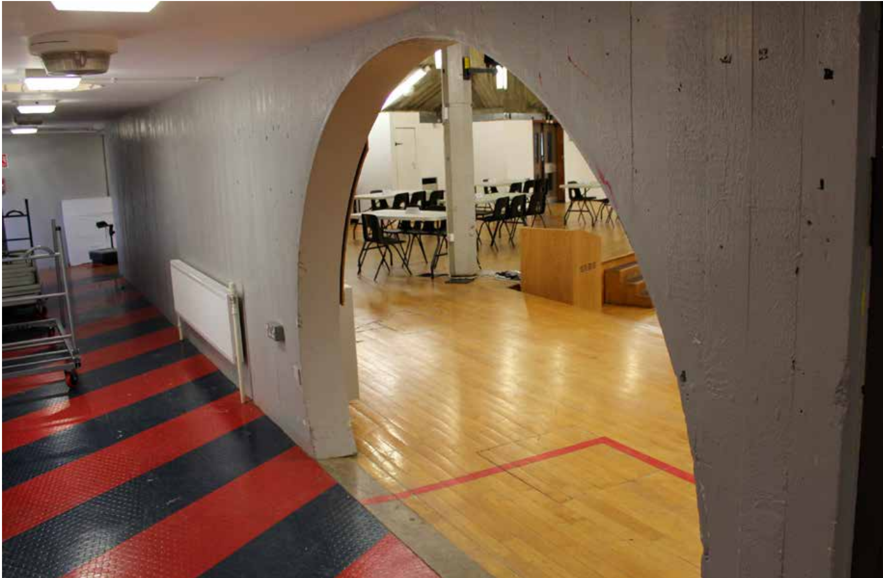
11.1 One of several circular apertures cut through the concrete wall of the assembly hall as part of the 'Schools for the future' pilot initiative.
