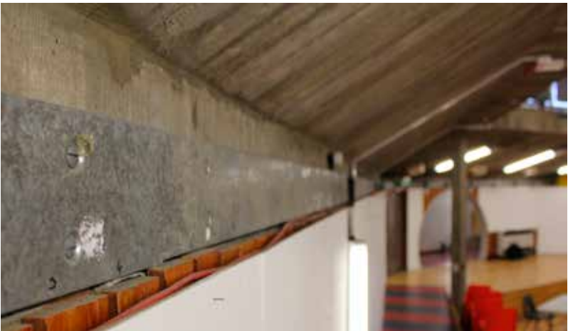
10.6 The original timber cladding to the internal periphery survives behind modern white boarding.
