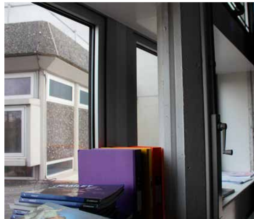
6.5 The distinctive double window design seen from inside a classroom. Although the original windows have been replaced, the original configuration and useful, deep cill remain.
