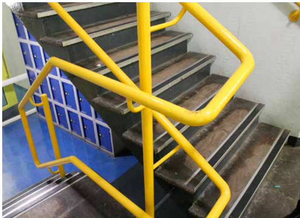
6.4 The original painted steel balustrade to each of the main stair towers.
