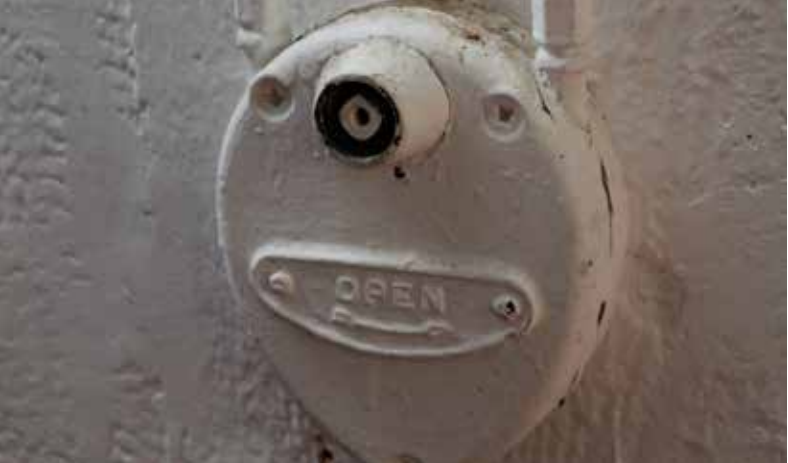
13.6 An original ventilator opener crank to operate the skylights above.
