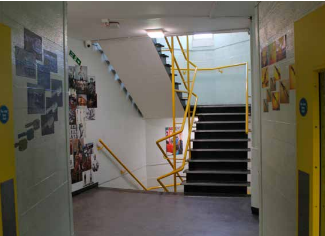
14.4 The painted steel balustrade and handrail to the stair cores is original to the building. These are to be retained and repainted where necessary.
