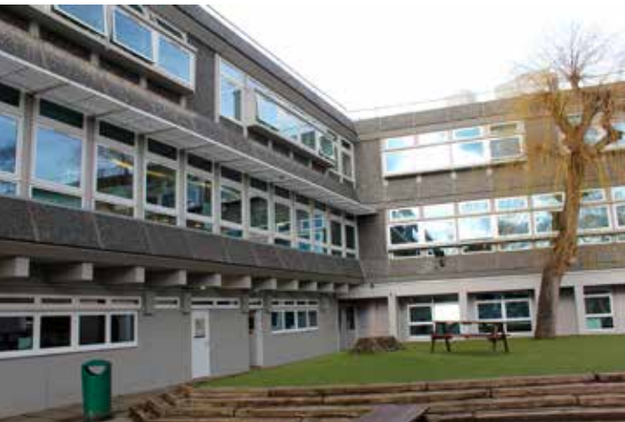
4.5 Existing main school building showing the recent replacement glazing, distinctive double layered windows (right) and iconic pre-cast concrete cladding units. Howell Killick, Partidge and Amis made excellent use of the expressive qualities of pre-cast concrete throughout their oeuvre.
