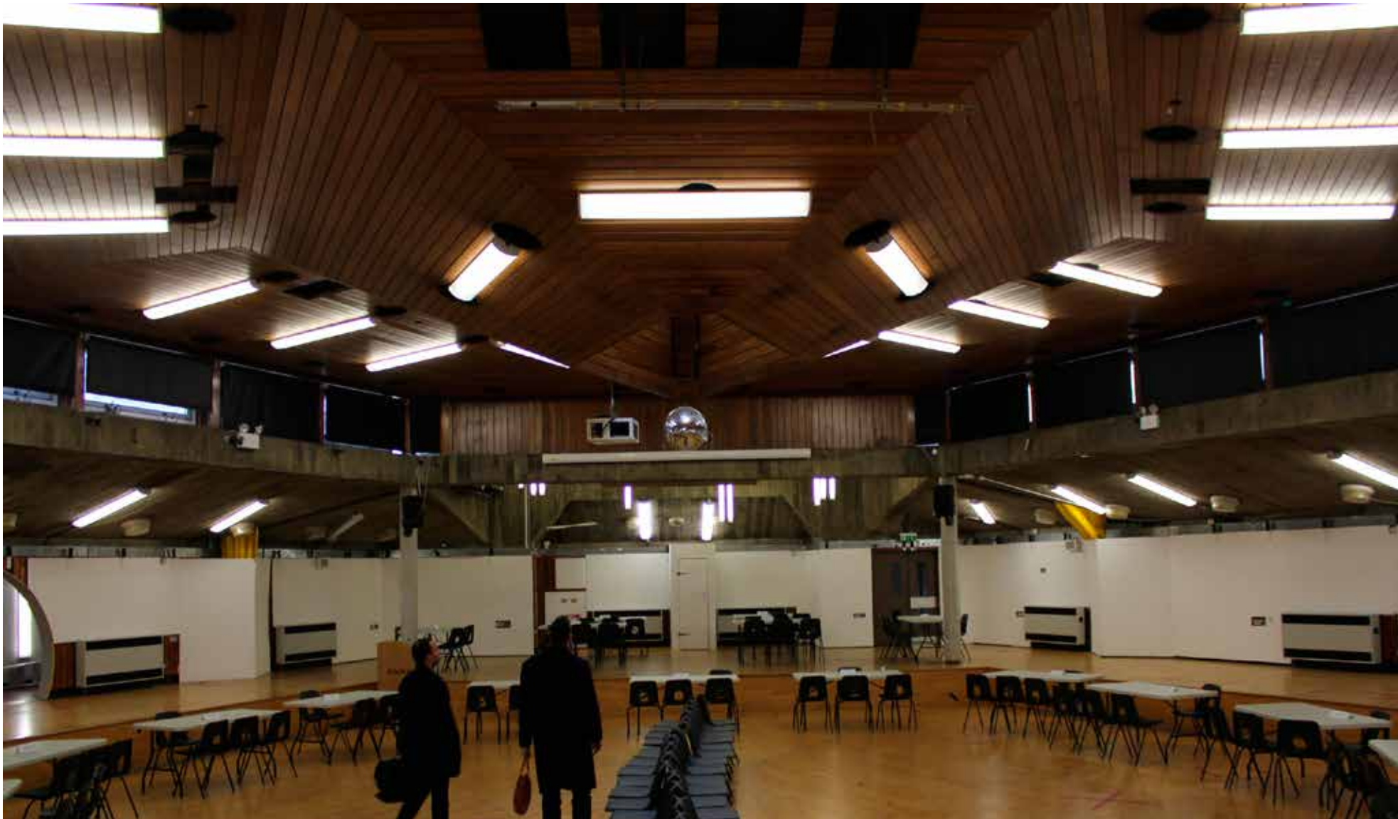
10.1 View of the main hall showing modern lighting and circular holes in the timber ceiling where the original light fittings have been removed. Note the clerestory glazing with modern blinds to the upper level and white boarding to the ground level, covering over the original timber cladding.
