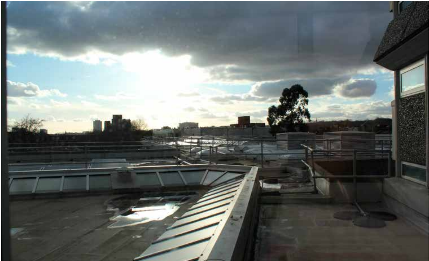
14.2 The flat roof deck above the art room with the continuous skylight to the periphery.
