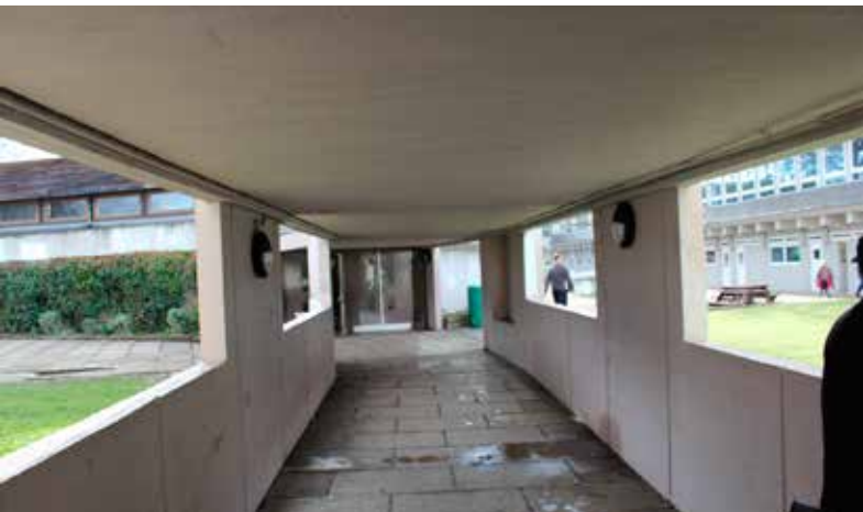
4.6 In-situ concrete covered walkway linking the main school building with the separate assembly hall.
