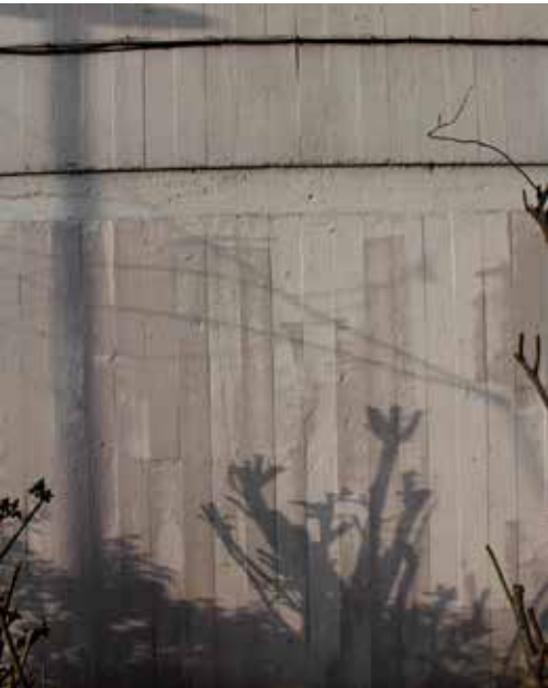
9.3 A detailed photo showing the timber shuttering imprint on the concrete elevations of the assembly hall.
