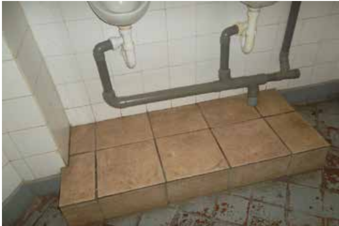
12.3 Modern plastic piping and plinth to the urinals in the boys toilet.
