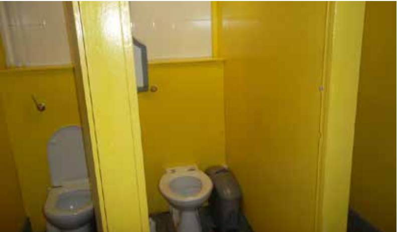
12.6 The original toilet cubicle partitions survive to both toilets. This photo shows an original style toilet to the right and a modern replacement to the left.
