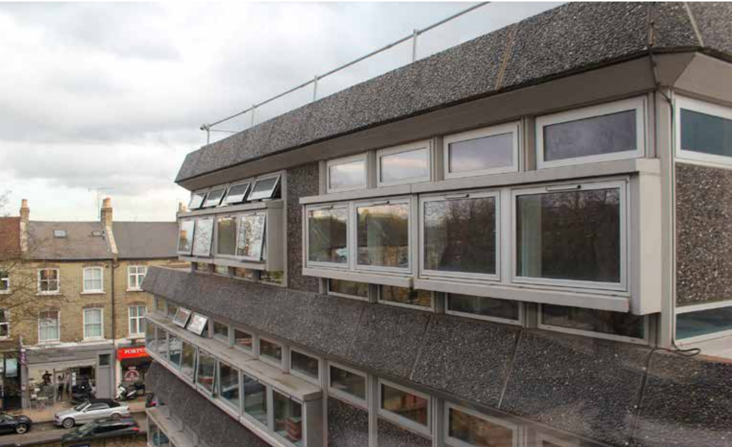
14.1 An external view of a series of classrooms in the main building. The original projecting services conduit, constructed from pre-cast concrete panels, still remains below the windows at each level. The services void cleverly conceals the hot water pipes that serve the classroom radiators, situated directly underneath the windows to the periphery.
