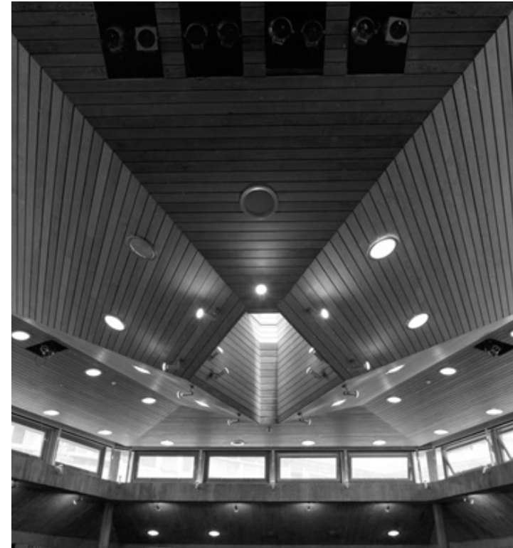
8.3 One of the dominant features of the assembly hall is the profiled timber ceiling and central skylight. Note the 4 apertures within the ceiling which allowed for studio lighting to be operated from within the void above.
