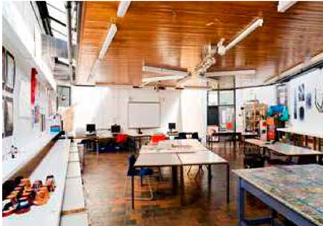
6.1 One of two art rooms with a glazed slot style skylight to the periphery of the original varnished timber ceiling.
