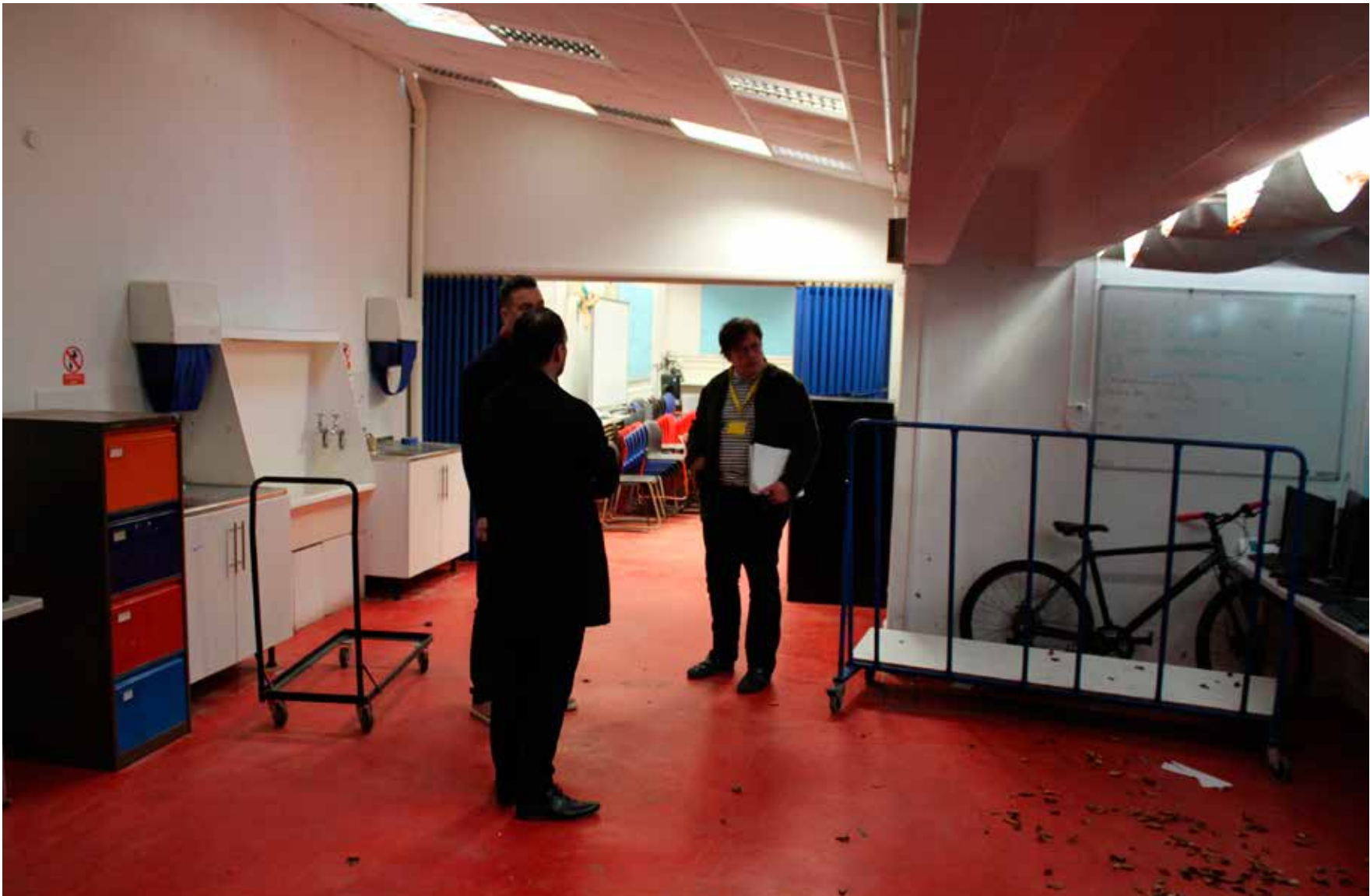
13.2 This photograph shows how the glazed roof is currently obscured by blinds, to the right of this image, and a suspended ceiling, to the left. The life expired glazed roof to this classroom is to be carefully replaced in its entirety.
