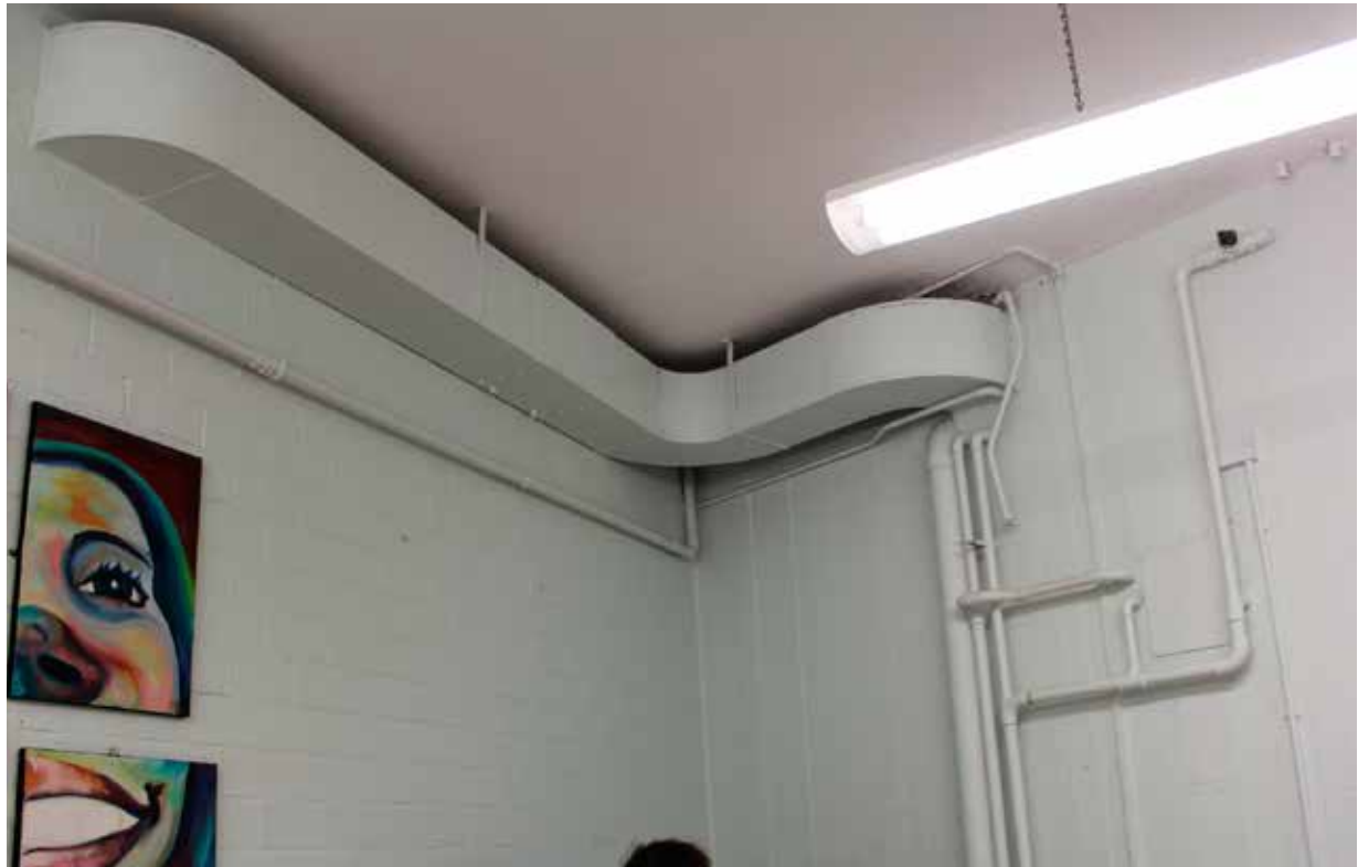
14.5 Existing surface mounted services conduits to a meeting room at ground level. Where new conduit / trunking is installed, these can be 'painted in' to match the wall finishes to minimise the visual intrusion.
