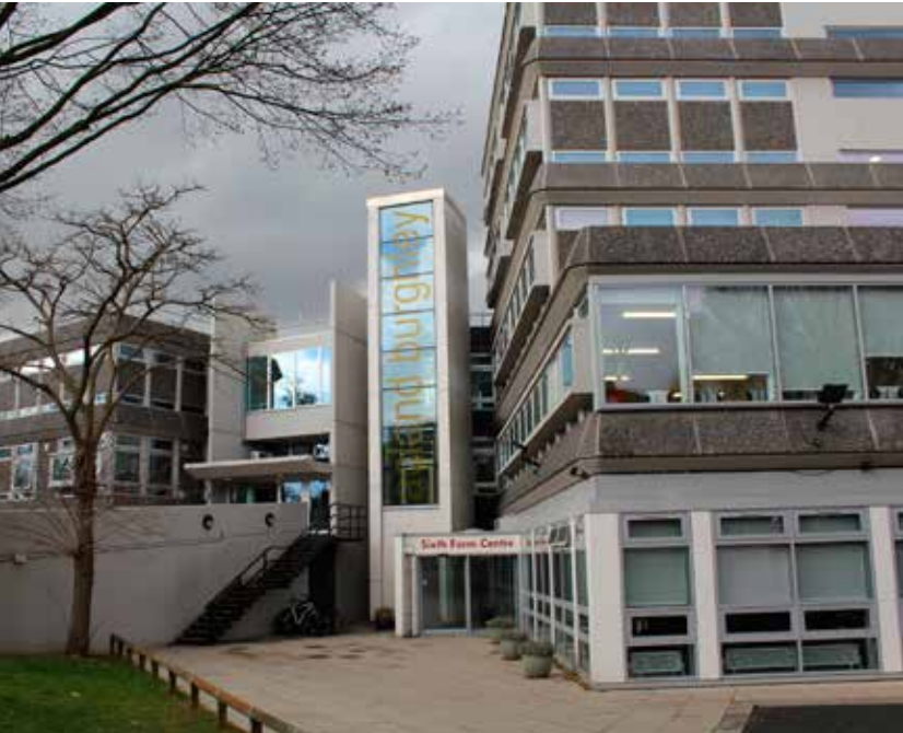
4.2 View from the south side lower level showing distinctive precast concrete cladding panels to the elevation and recent replacement aluminium windows to the main school building.
