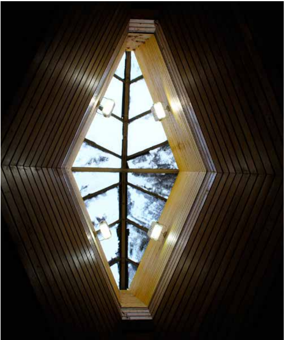
10.2 The central lantern to the assembly hall roof currently leaks and is in need of attention.
