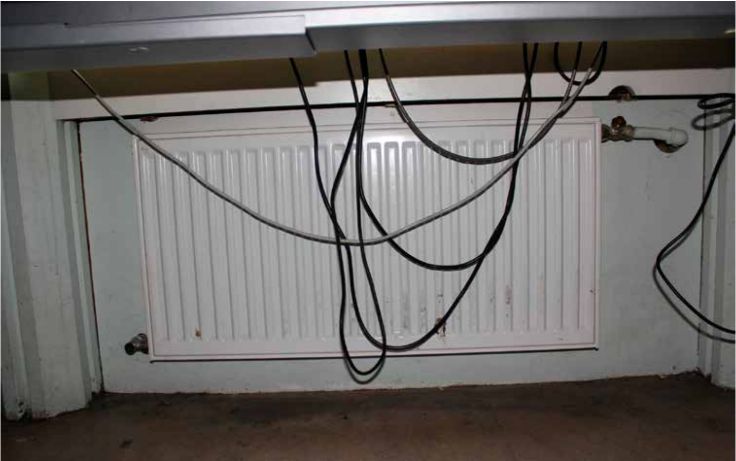
15.5 A typical classroom radiator with concealed pipework to the rear. The existing painted timber board is to be upgraded with a new fire rated Supalux cladding panel. The proposed improvements can help with cable management.
