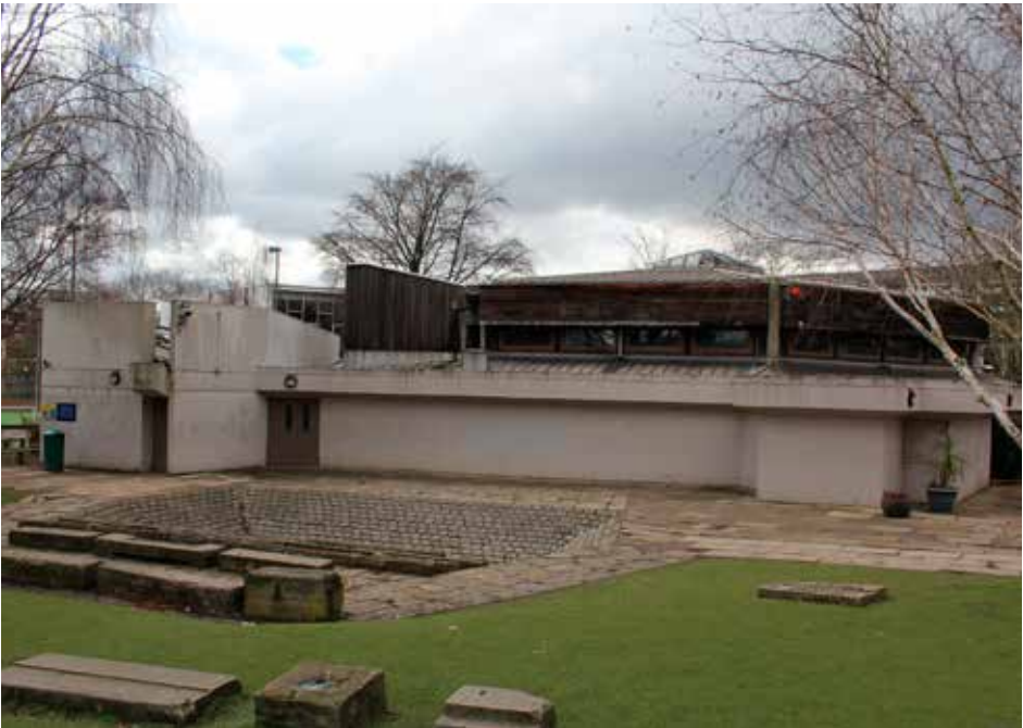
4.3 External view of the auditorium. Note the central glazed skylight, Standing seam aluminium roof, timber cladding and original timber clerestory windows to the upper level. In-situ concrete walls form a sturdy base element.
