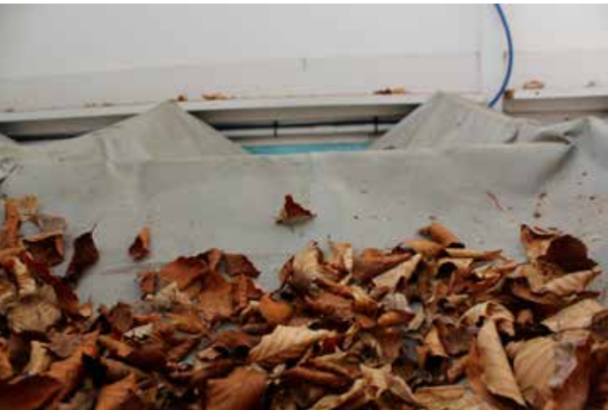
13.5 A collection of leaves on top of the sun blinds caused by damaged skylights.
