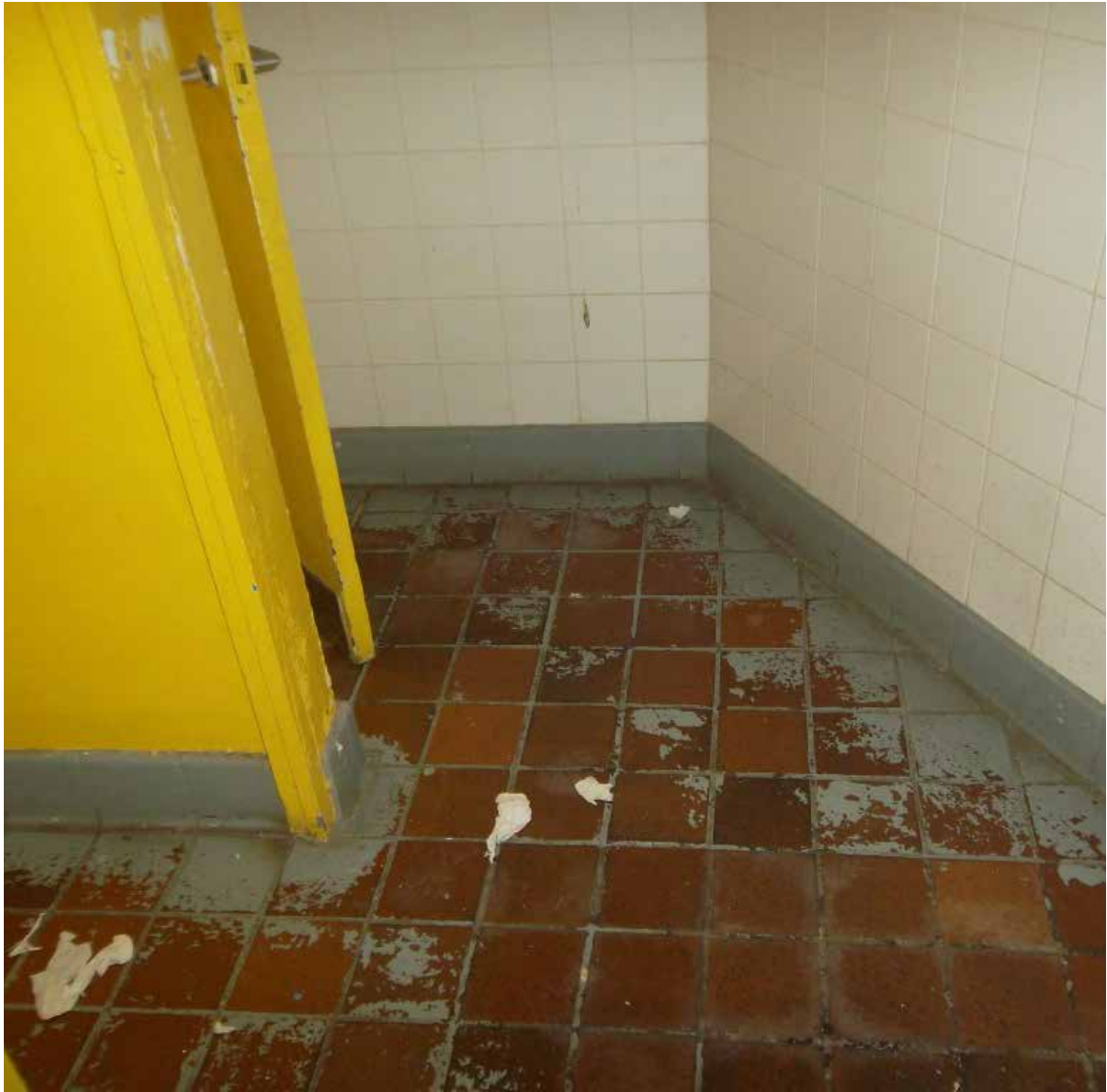
12.2 The original quarry tiled floor is intact to both toilets. These could be cleaned of paint and retained as a heritage feature.
