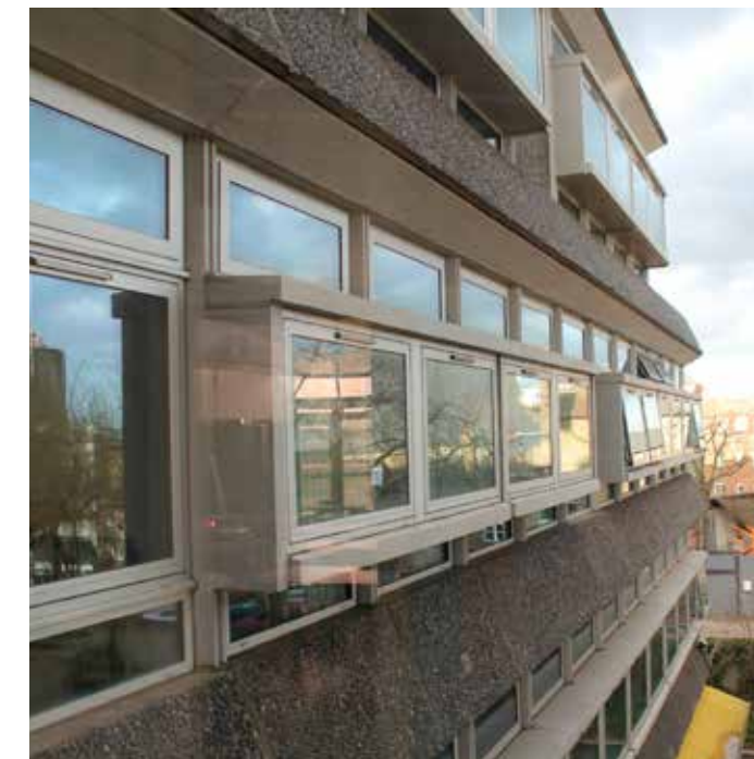
6.6 The double window design seen from the exterior. The original projecting service conduit still remains below the windows at each level. This technical drawing ( above right ) shows how the hot water pipes to serve the radiators were cleverly concealed in this purpose designed feature. For full technical drawing see appendix 2.
