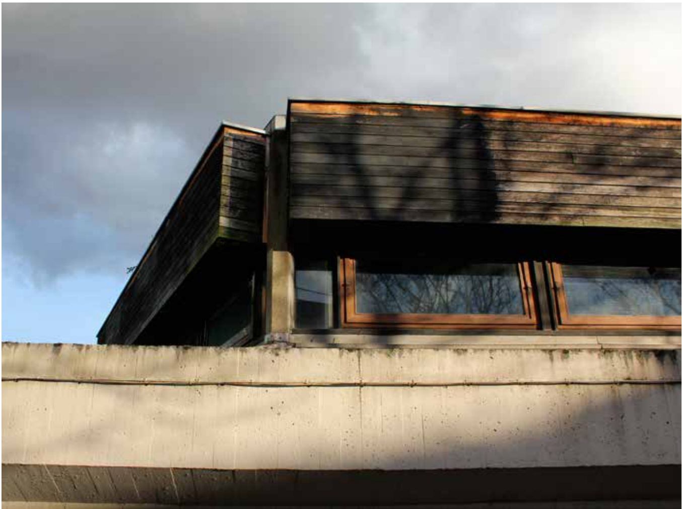
9.2 This photograph shows the timber cladding to the upper part of the assembly hall. The original boarding is heavily weathered and in need of refurbishment. The original timber windows with metal brackets are also in need of a careful restoration but do not appear in too bad a condition.
