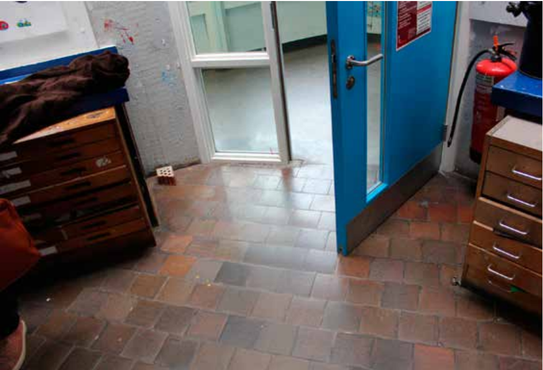
15.3 The original quarry tiled floor to the art room. These tiles are to be cleaned and retained where possible throughout the building and celebrated as an attractive heritage feature.
