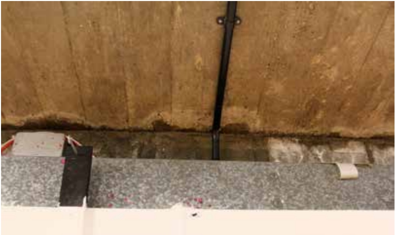
11.6 Signs of damp to the south-east side of the hall at ceiling level.
