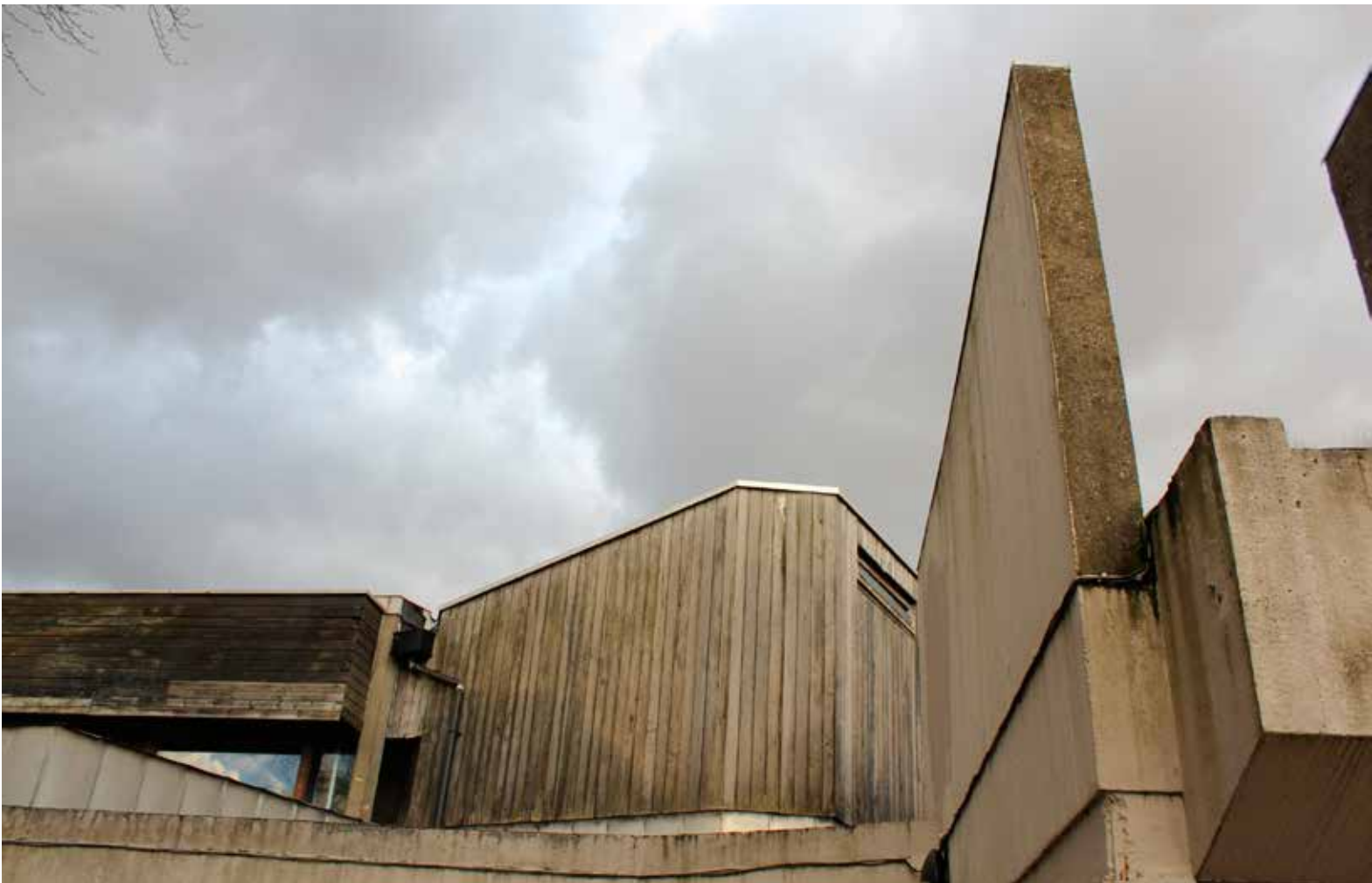
9.1 An external view of the assembly hall upper level. Visible is the simple palette of materials used throughout the building; concrete, timber, glass and aluminium. The distinctive timber-clad form in the centre of this image is the flytower, over the main stage area.
