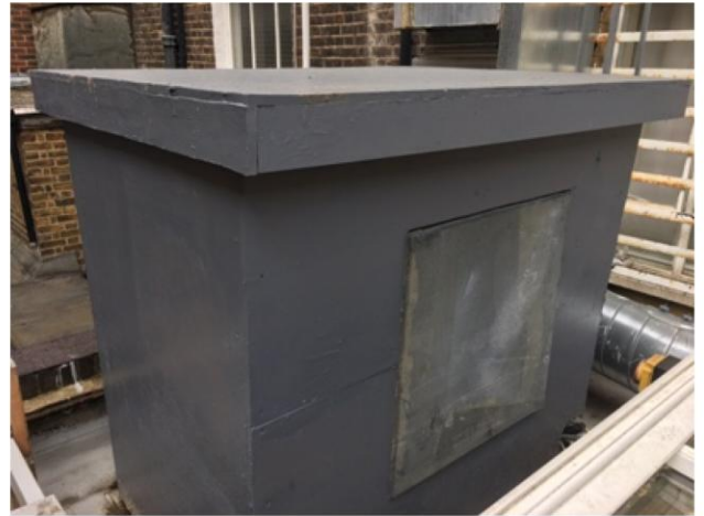
View of acoustic enclosure around large chiller unit on roof.
