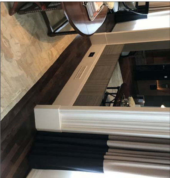
R130 SITTING ROOM NTF06, DINING ROOM NTF06 Showing new joinery to house curtains tracks
