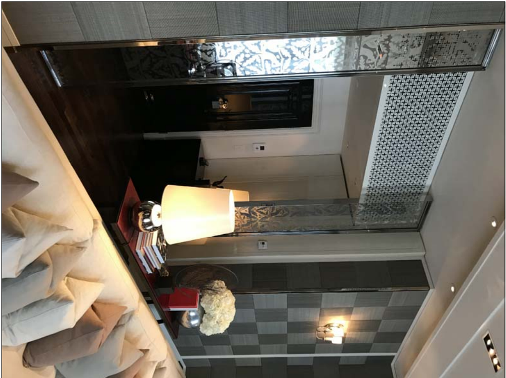
R127 LOBBY NTF17 Showing new decorative A/C grills and mirror fronts for cupboards
