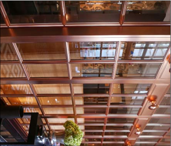
R124 MASTER BEDROOM LOBBY NTF04 Showing new copper plated glass paneling, door and partition
