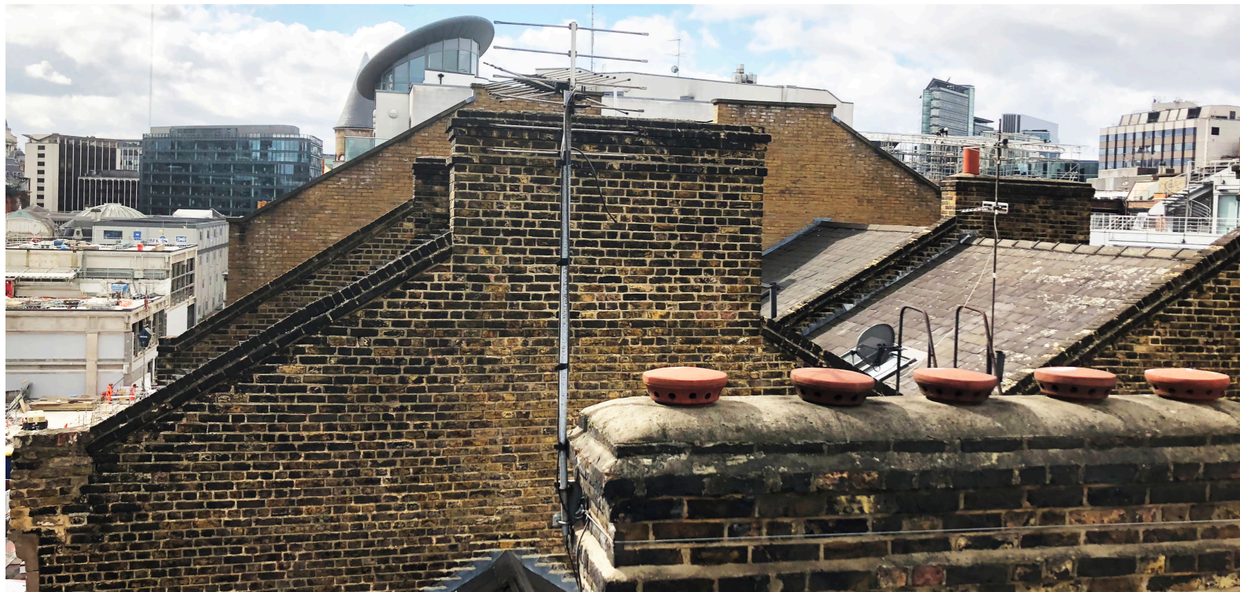
View of neighbouring flank walls at roof level.
